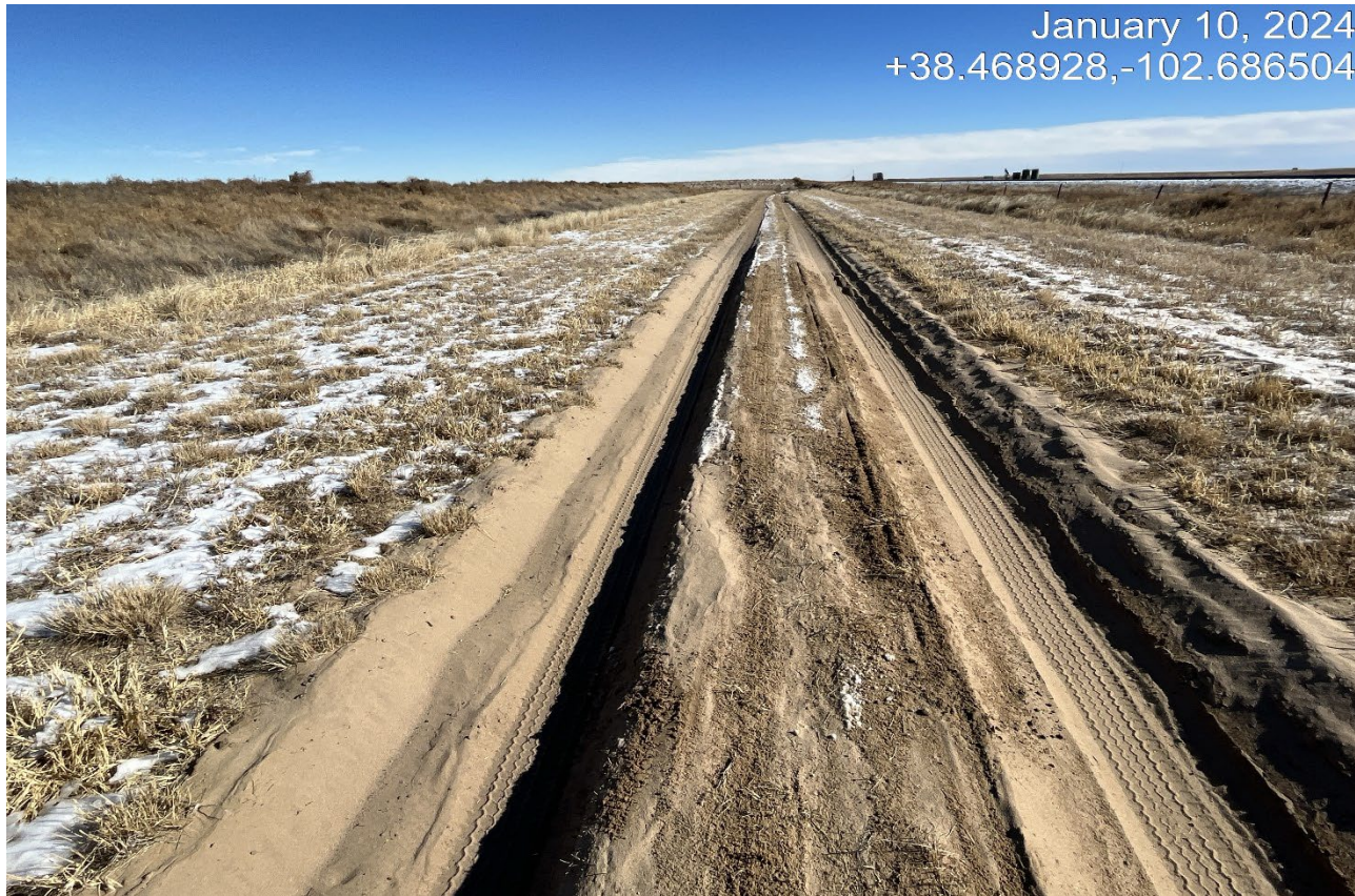
Photo 1. Facing east along the access road. There is deep ruts along this area of the road which is not stabilized.
