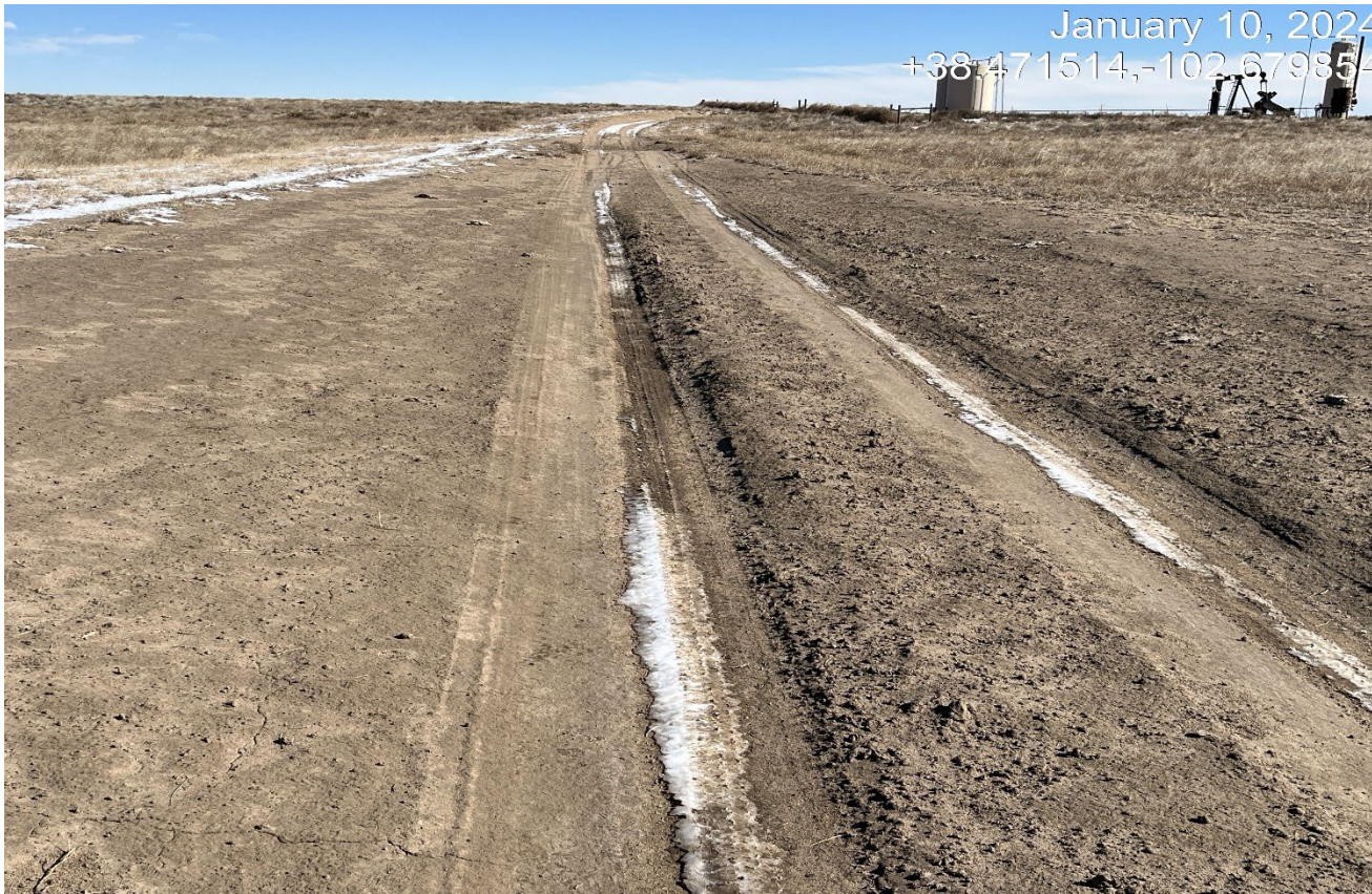
Photo 2. Facing east along the road near the location. This area is swalled and the road has been widened due to vehicle driving avoid this area during wet conditions..
