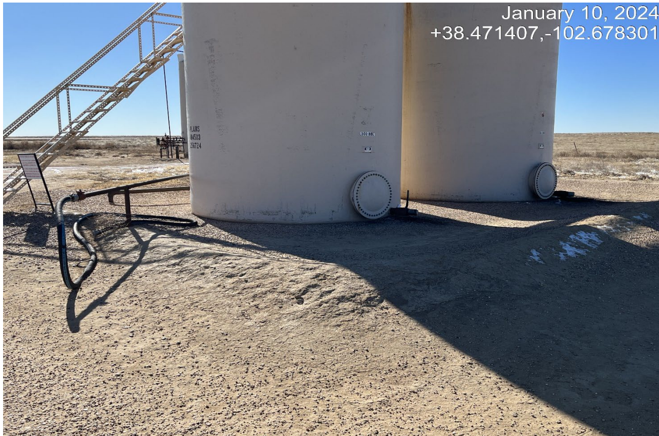
Photo 5. The berm around the tanks are inadequate to contain a spill.
