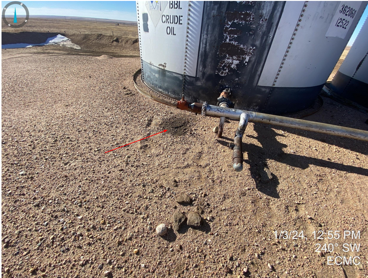
Photo 6. Stained soil observed near the connection/loadout lines at the tank battery.
