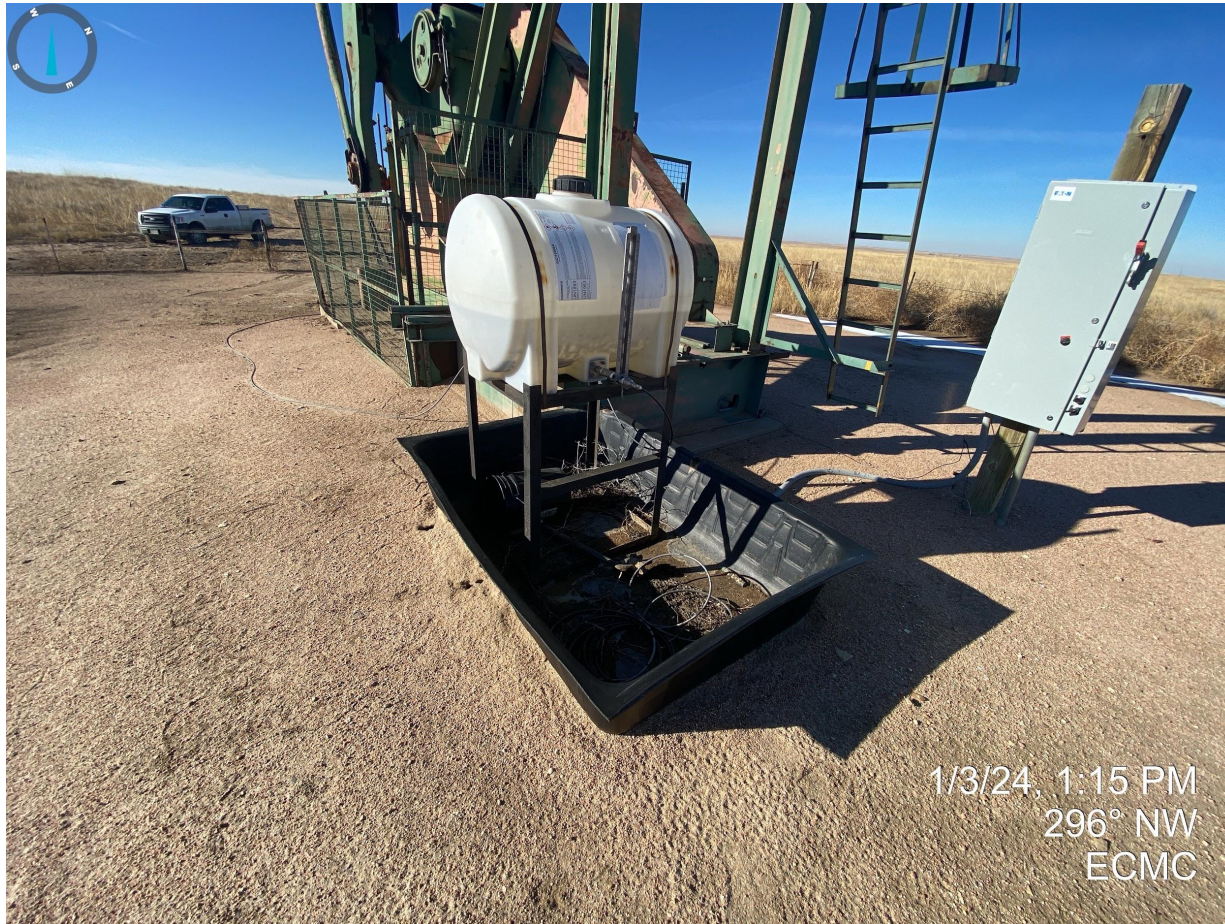
Photo 24. No wildlife exclusion equipment observed at day tank secondary containment.
