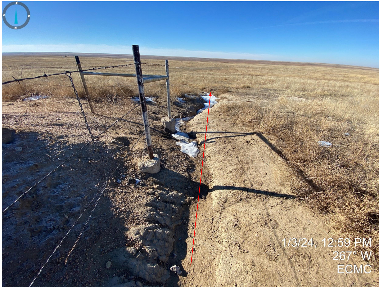
Photo 9. Erosion degradation (e.g. gully) occurring on the northwestern portion of the tank battery. No apparent stormwater control measures observed during this inspection.
