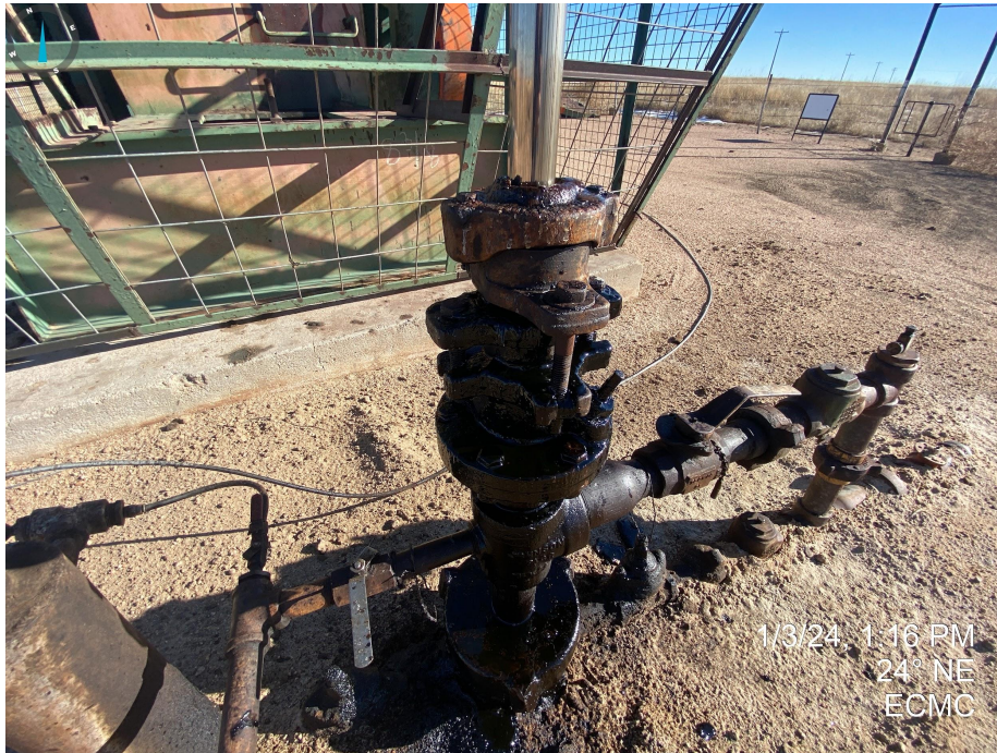
Photo 26. Stained soil and visible leak at wellhead.
