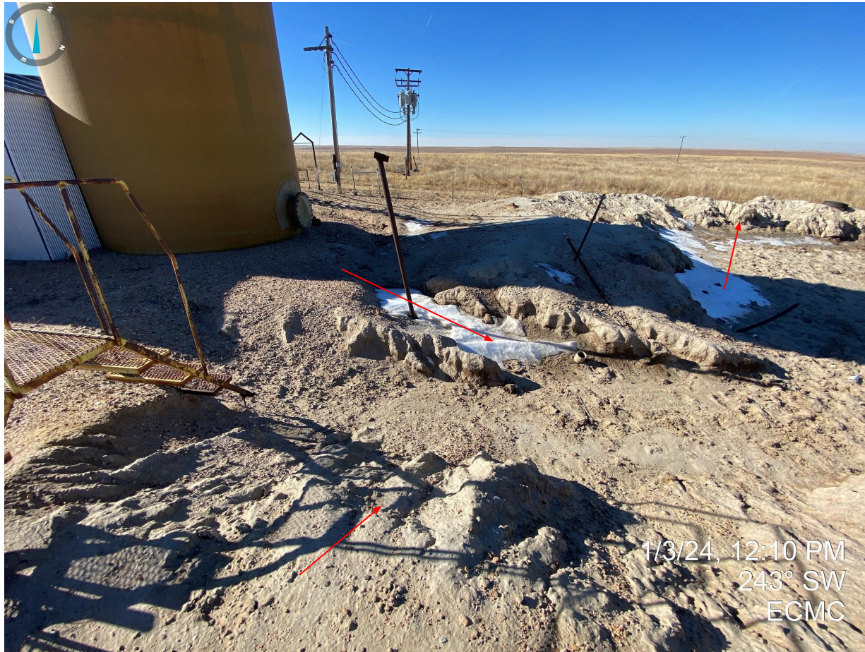
Photo 4. Erosion degradation occurring on pit berms.
