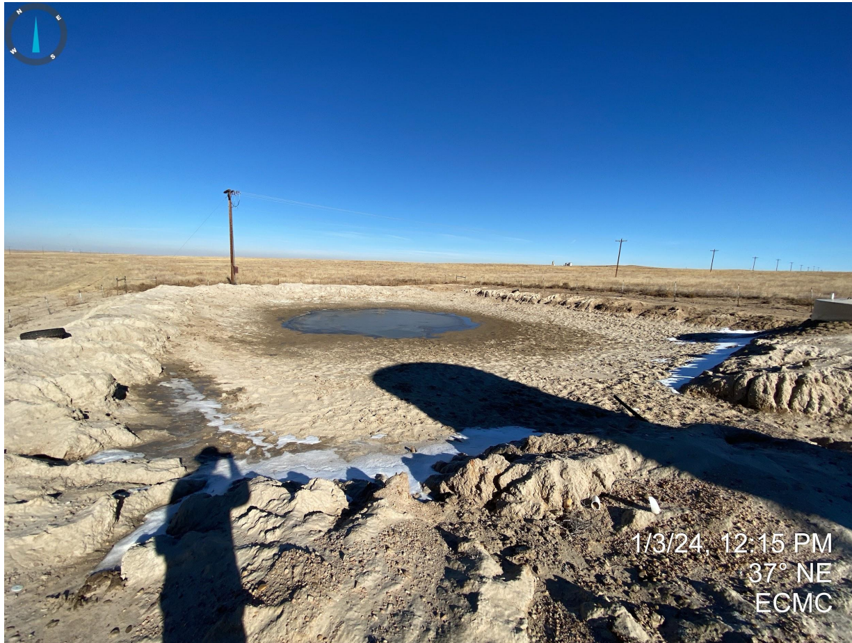
Photo 12. Overview of pit from the southwest corner. The pit is experiencing severe erosion degradation.
