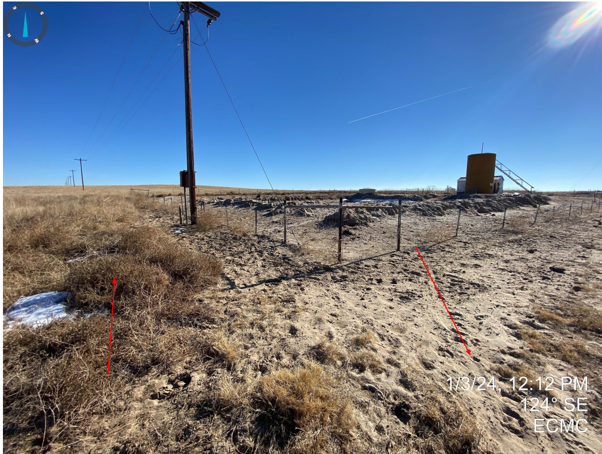
Photo 9. Taken from the northwest corner of the pit. Photo illustrates no apparent stormwater controls that would prevent the sediment transport (pictured by red arrow) from leaving the location. Additional stormwater controls are needed for the location. Also pictured, undesirable vegetation (russian thistle).
