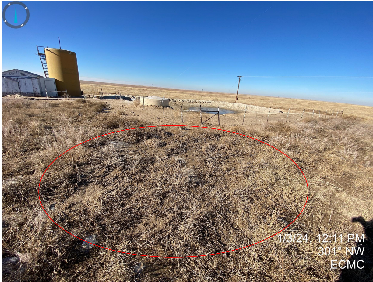
Photo 6. Taken southeast from the pit. Blow sand accumulations were observed southeast of the pit, indicating wind erosion from unstabilized production areas.
