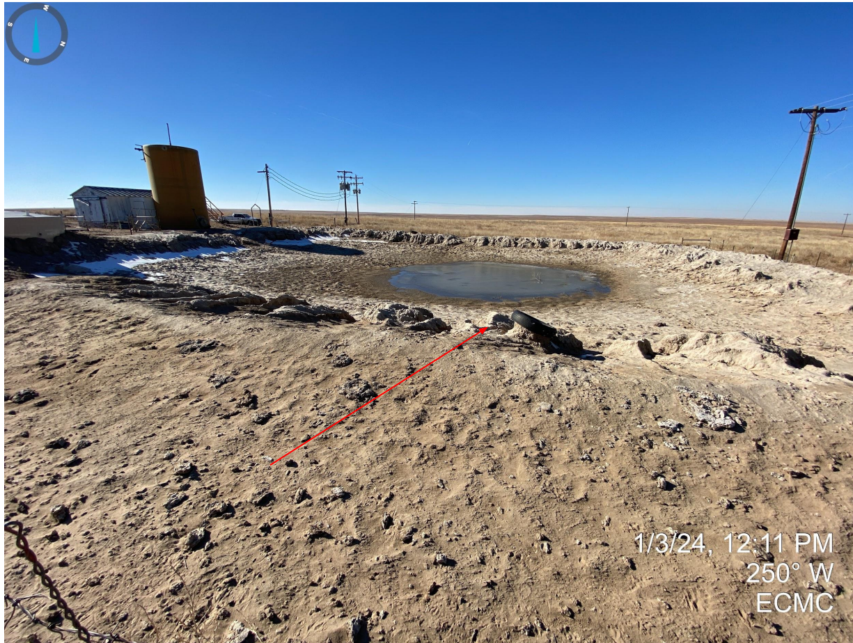
Photo 7. Taken from the east side of the pit. Photo illustrates that pit berms are eroding and the production areas are not properly stabilized.
