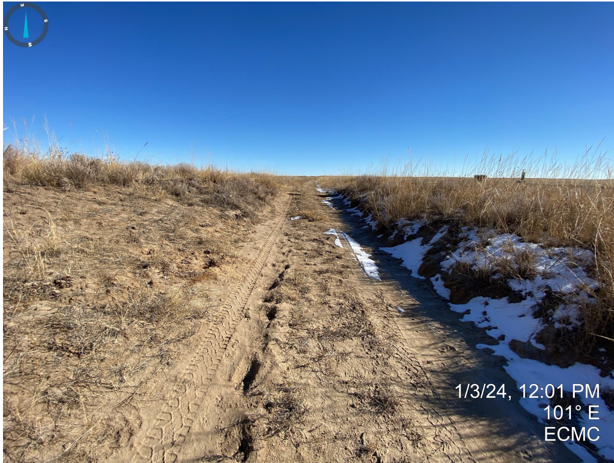
Photo 1. Taken from the eastern portion of the access road, facing east. The access roads do not appear to have been reclaimed as they are not contoured/graded to reflect pre-disturbance/reference area topography. Additional reclamation activities are required.
