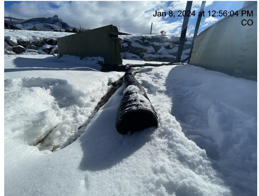
Photo # 2037 Flowline heating insulation open ended
