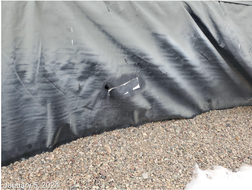
Photo 8: Photos examples showing holes observed within the liner at the tank battery.
