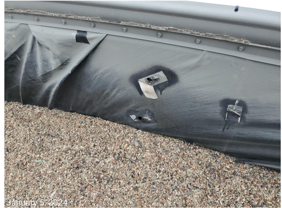
Photo 8: Photos examples showing holes observed within the liner at the tank battery.
