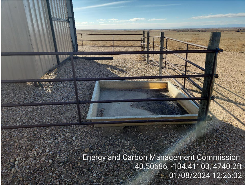
Photo 3 – Unused Secondary Containment
