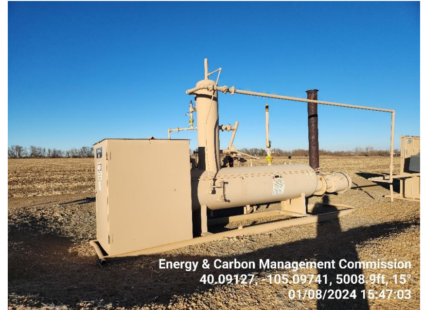
Photo 6 Horizontal Heated Separator.
