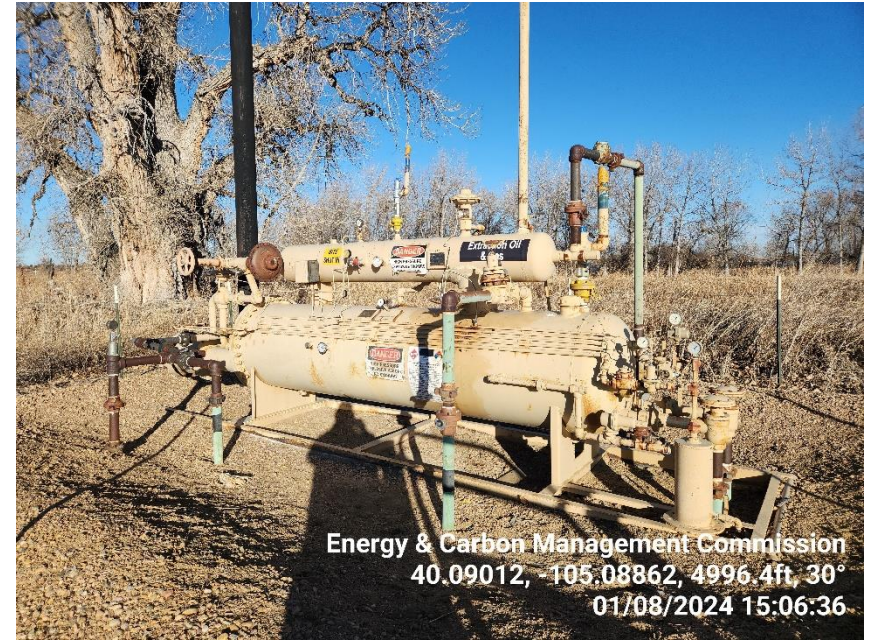
Photo 6 Horizontal Heated Separator.
