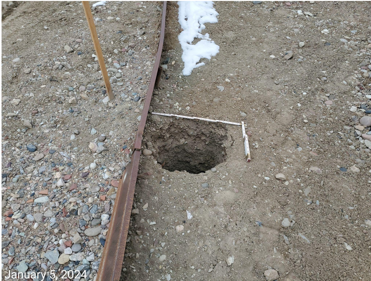
Photo 4: Photo taken from the separator equipment on the east end of the Location. Photo shows sinkhole. Sinkhole is ~1.5' wide and 2.5' deep.
