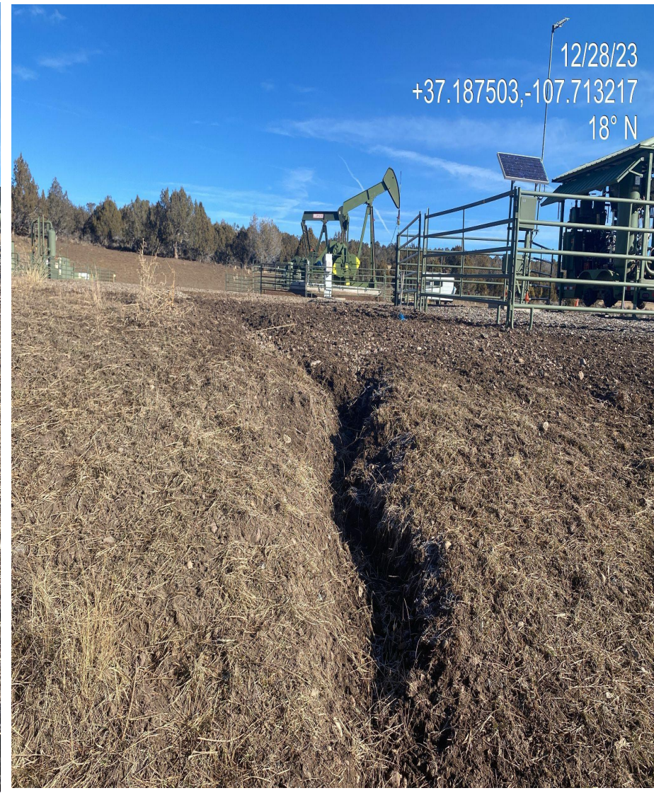
Photo 2. View of gully erosion forming in the southern edge of the disturbance.
