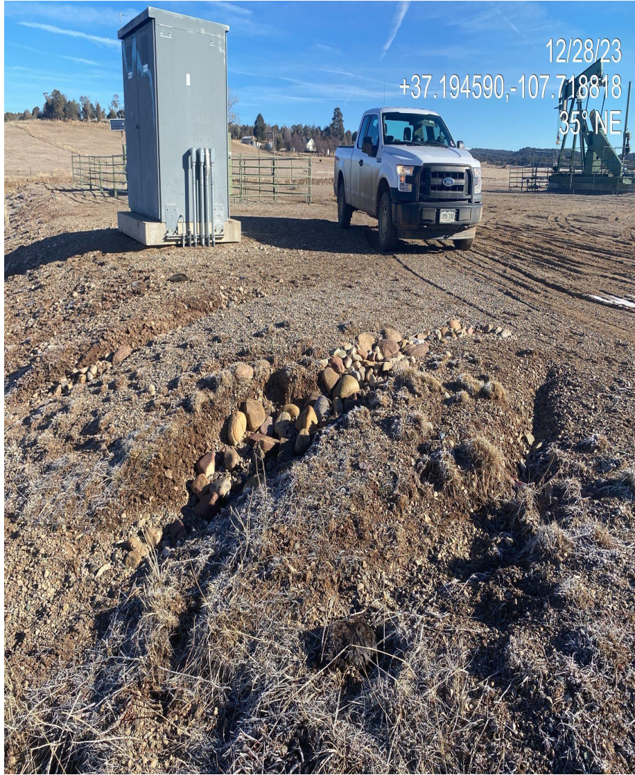
Photo 2. View of rill/gully erosion forming on the western edge of the disturbance. Current round river rock stormwater BMPs are not adequate.
