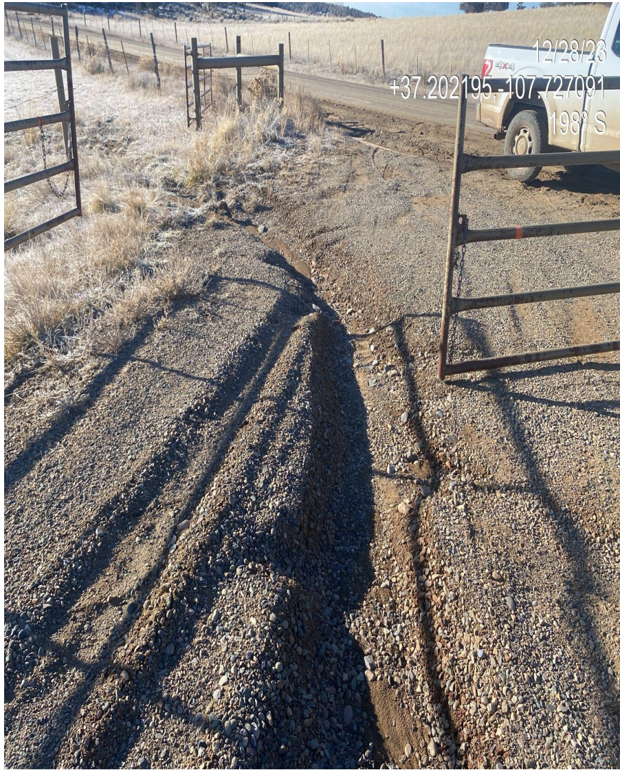
Photo 2. View of rill/gully erosion forming at the access point.
