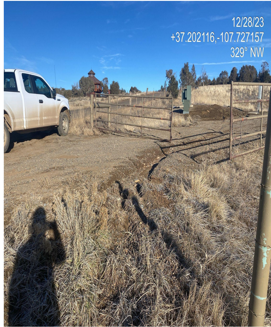
Photo 2. View of rill/gully erosion forming at the access point.
