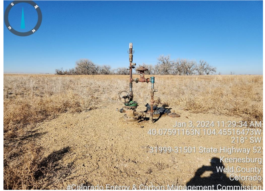
Photo 2 Well head. No sign DEAD WEEDS DEBRIS
