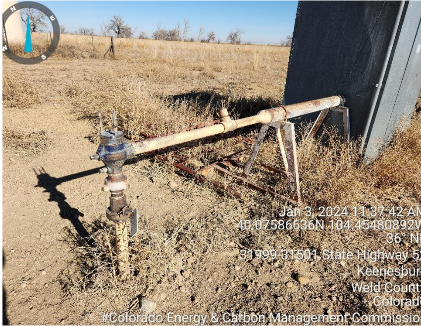
Photo 9 Meter tube LOTO and pined pulled.
