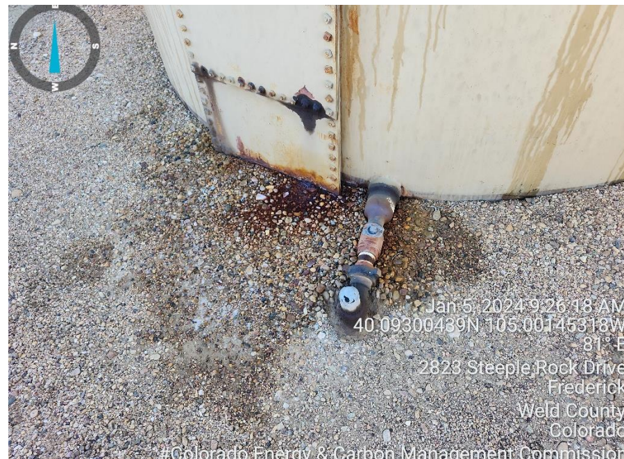
Photo 12 Crude oil tank stained soil and what appears to be mechanical issues with the 2 in piping and rusted bolts on inspection hatch.
