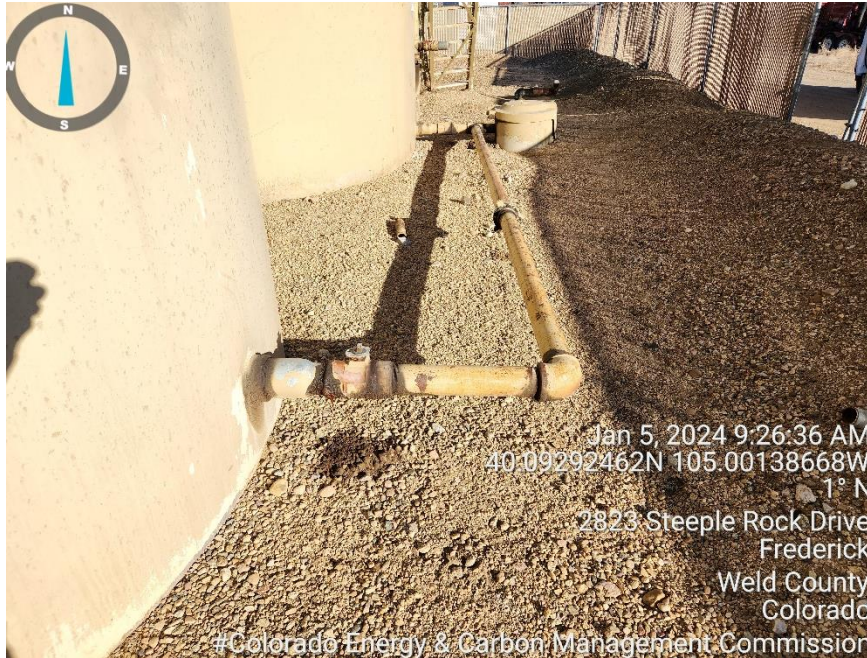
Photo13 stained soil under crude oil load out lines and what appears to be mechanical issue with 2 in piping
