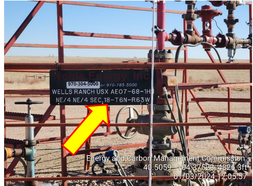
Photo 6 – Wrong Section 18 on Wellhead Signs
