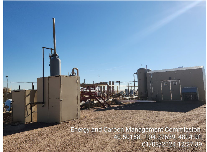
Photo 10 – Instrumental Air Unit
