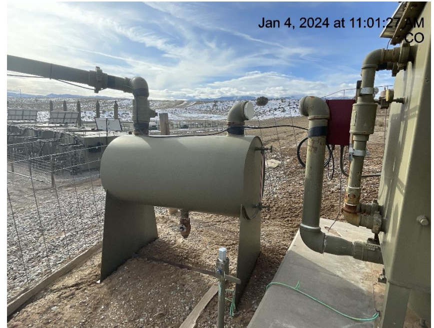
Photo # 1728 Unused equipment – ECD disconnected
