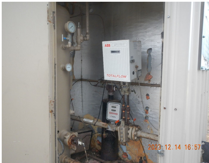
5. Digital gas meter run and vertical separator inside meter shed.
