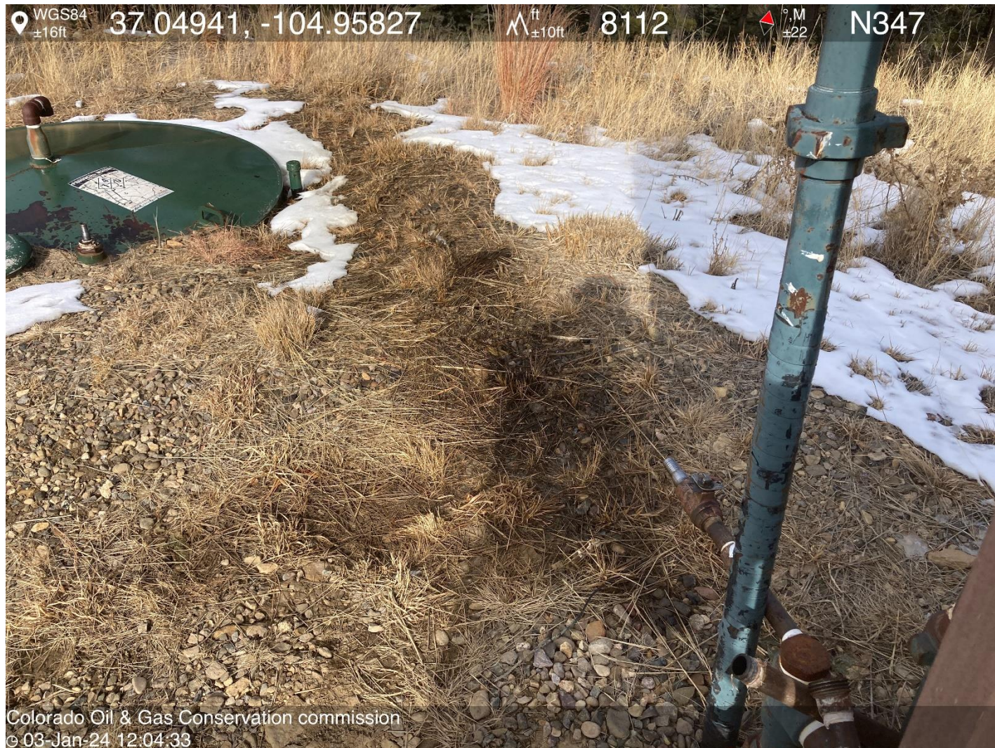
PHOTO 4: AREA OF IMPACTED SOIL APPEARS TO BE FROM SEPARATOR DRAIN (APPEARS THAT HOSE CONNECTING SEPARTAOR DRAIN TO 25 BBL TANK WAS REMOVED). DISCONTINUE DRAINING SEPARATOR IN GROUND, Conduct maintenance on equipment, cleanup stained material and review self inspection processes. COMPLY WITH RULE 1002,(2).D. CA DATE 2-3-2024.
