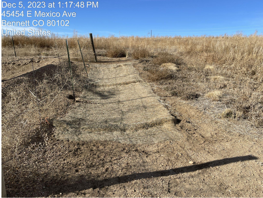
Photo 5. Photo taken of erosion control blankets, vegetation and weeds (Russian thistle) in interim reclaimed area. Photo taken facing northwest.
