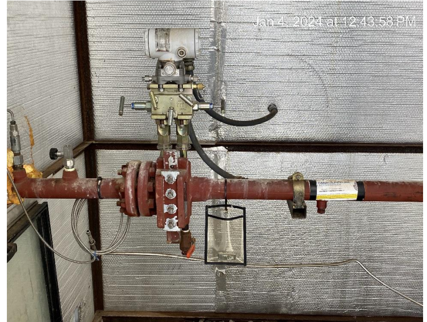
No visible display of gas meter calibration
