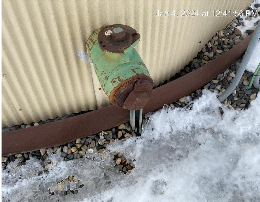
Cracked loadline plug
