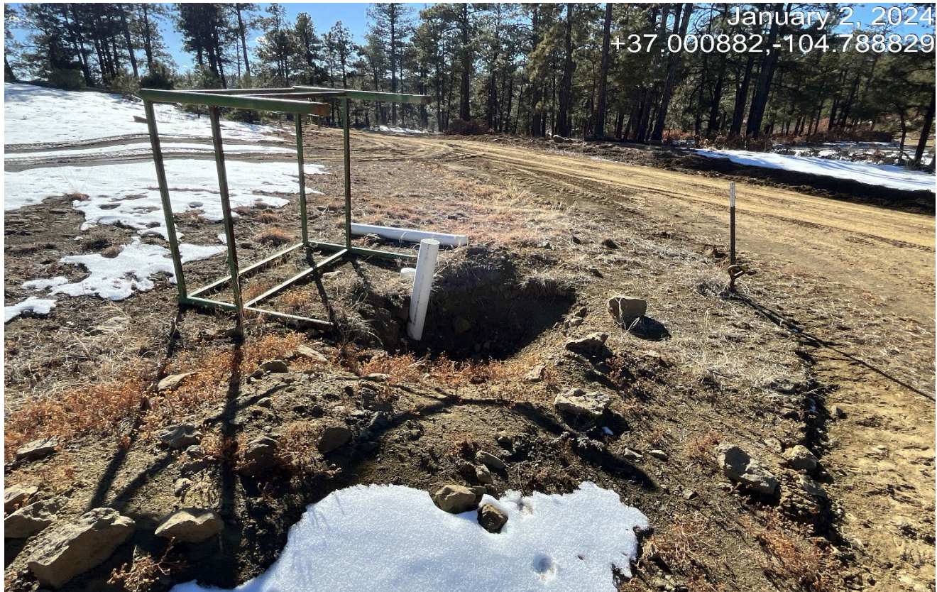
Photo 8. The plastic pipe has been excavated and pipe fence guard is not in place. .
