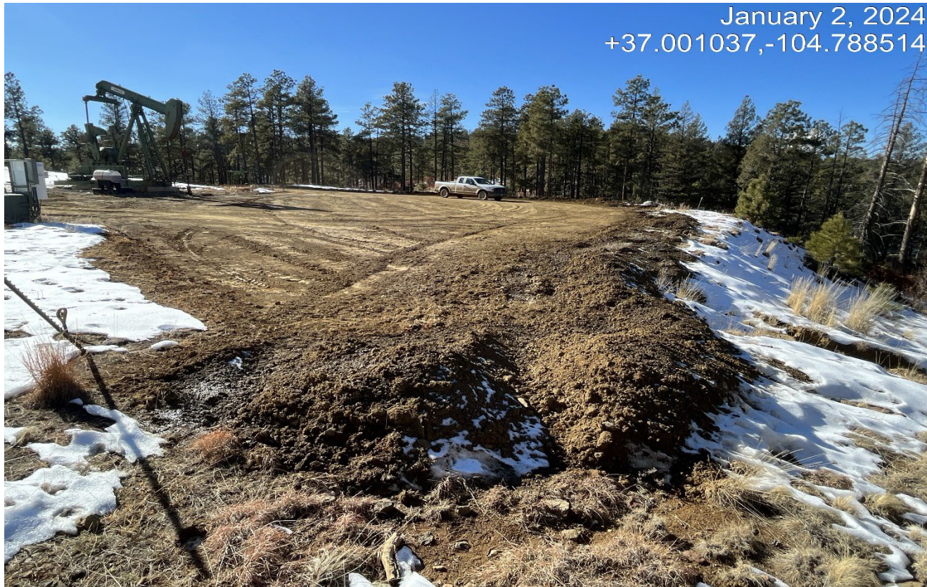
Photo 7. Northeast corner of the location. Soil has been pushed out from snow removal and will need to be replaced. Disturbance area will need to be reclaimed.
