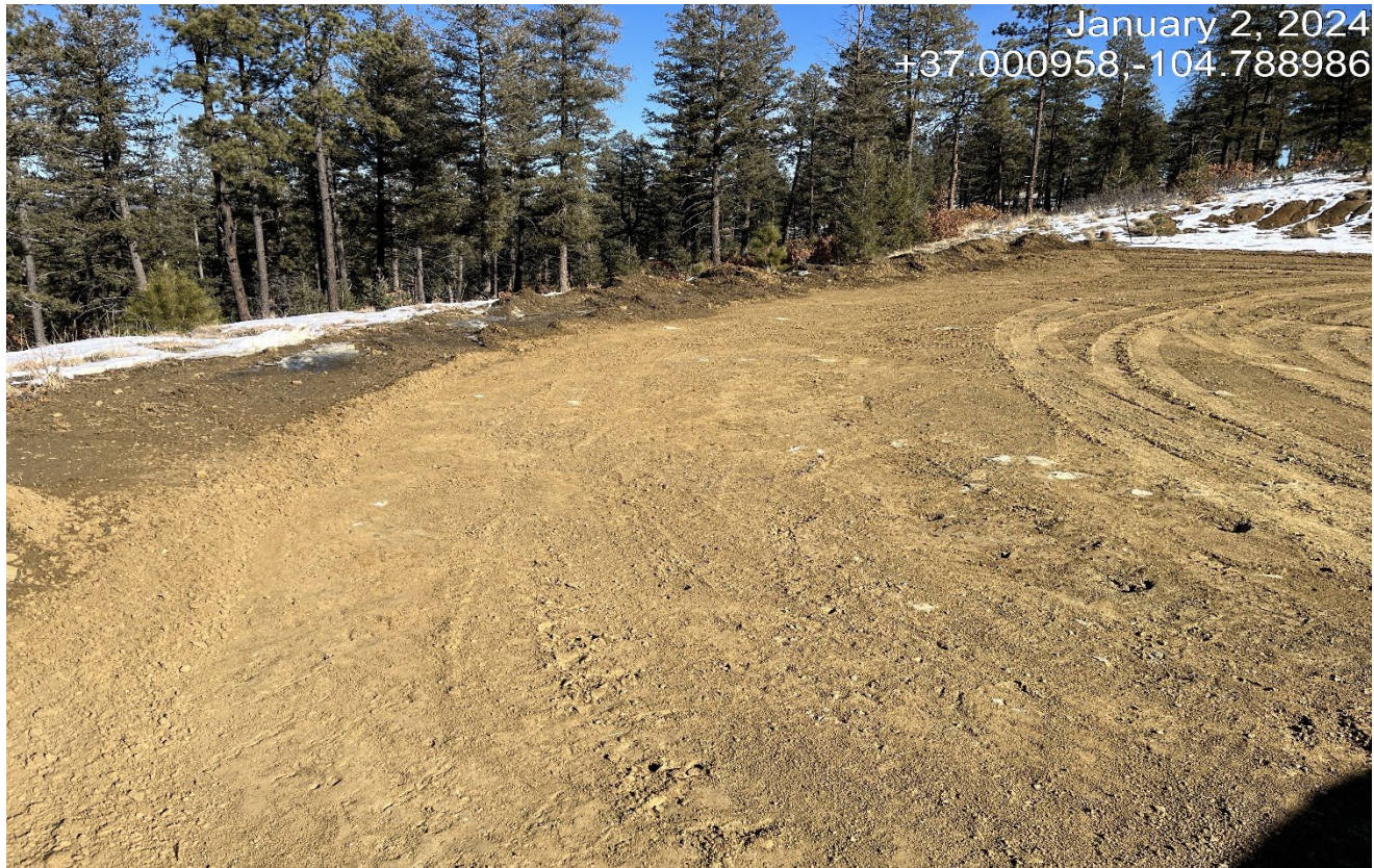
Photo 2. Facing toward north side of the location. This area has been graded and soil is pushed out to the edge. This interim area will need to be reclaimed.
