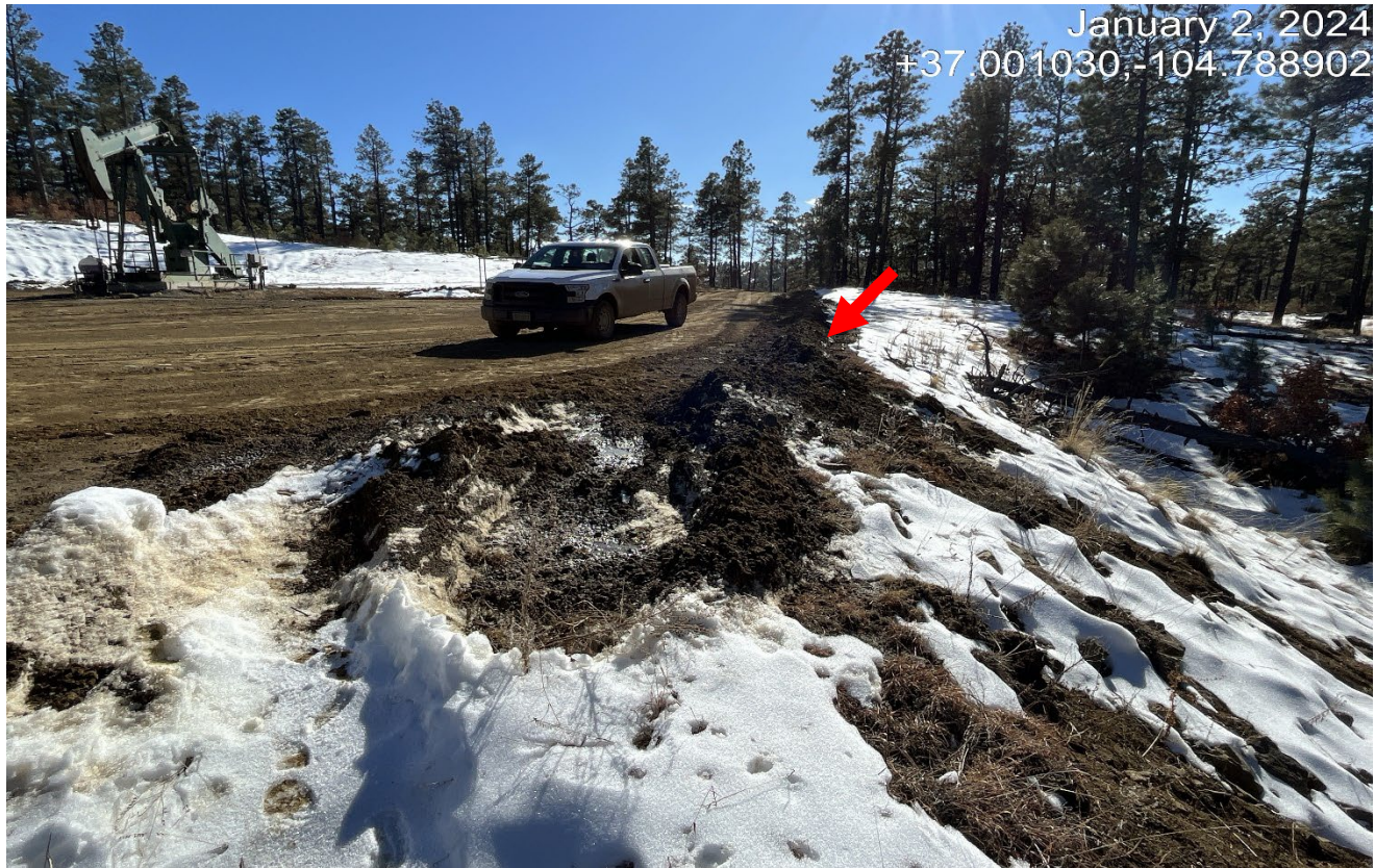
Photo 3. Facing south at the west side of the location. Soil has been pushed out along the edge and will need to be pulled back..
