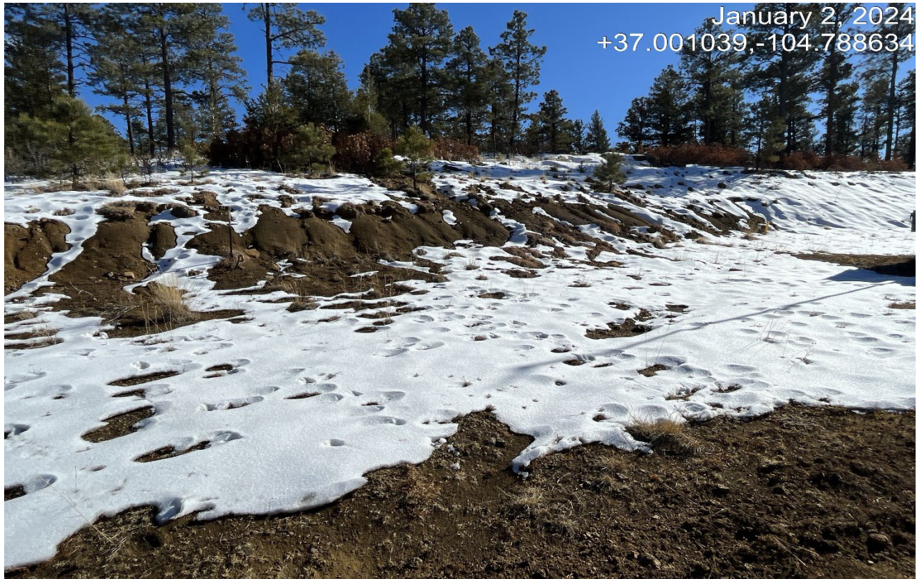
Photo 6. Facing toward the cut slope which has sign of erosion that need to be repaired..
