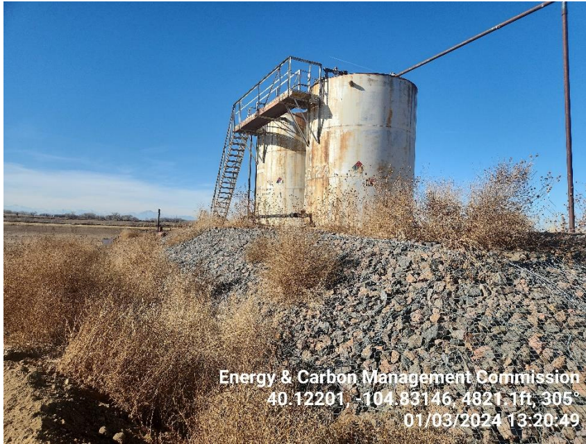
Photo 21 TB berm is overrun with dead undesirable vegetation.
