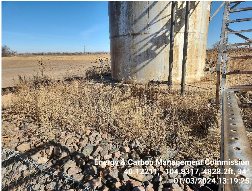
Photo 17 TB berm is overrun with dead undesirable vegetation.
