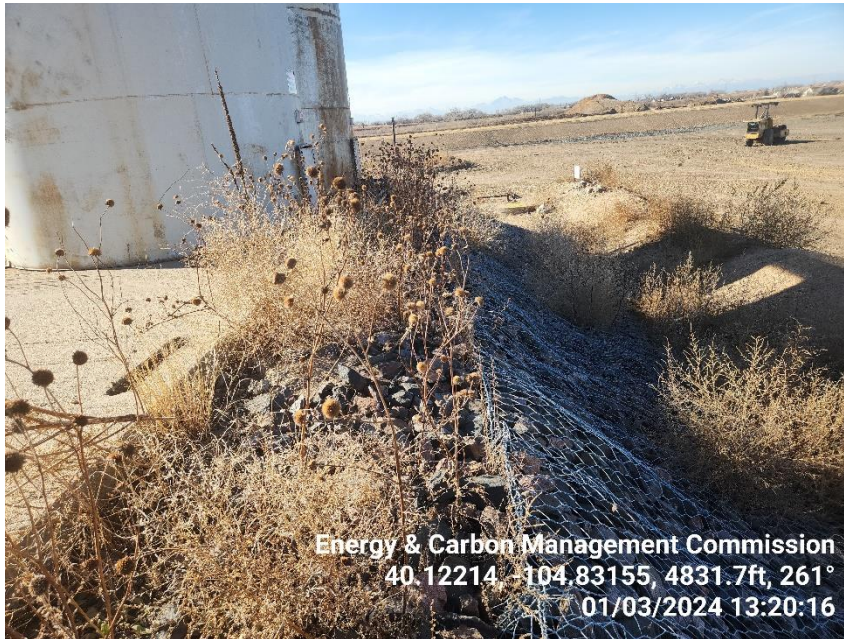
Photo 19 TB berm is overrun with dead undesirable vegetation.
