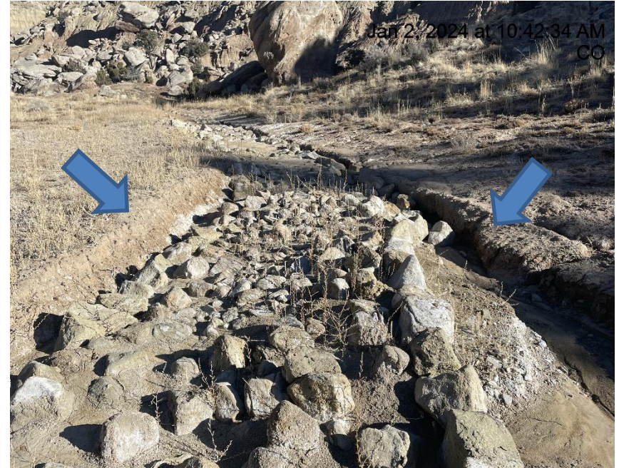
Photo # 1390 Rip Rap Run needs maintenance, stormwater has eroded around both sides of BMP & there's sediment buildup in some areas of BMP (eastern side of location)
