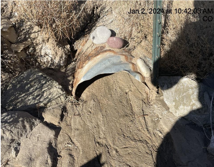
Photo # 1389 Culvert at entrance to location needs maintenance
