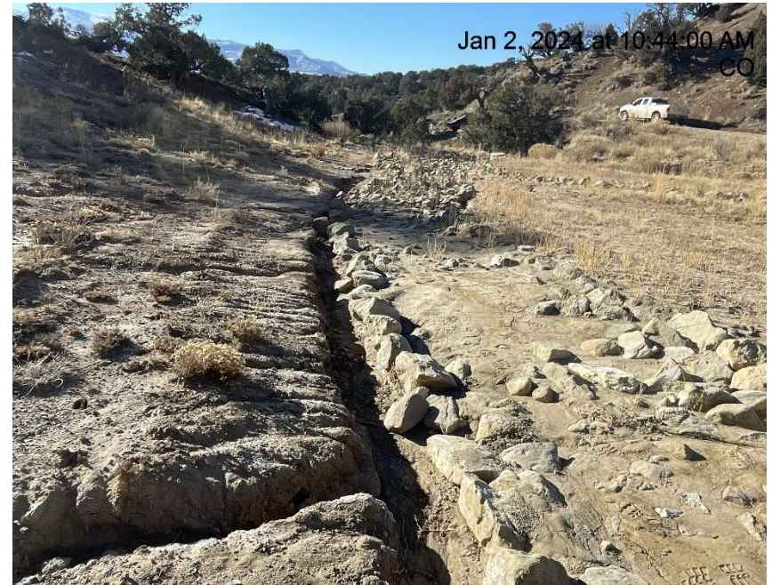
Photo # 1392 Rip Rap Run needs maintenance (eastern side of location)
