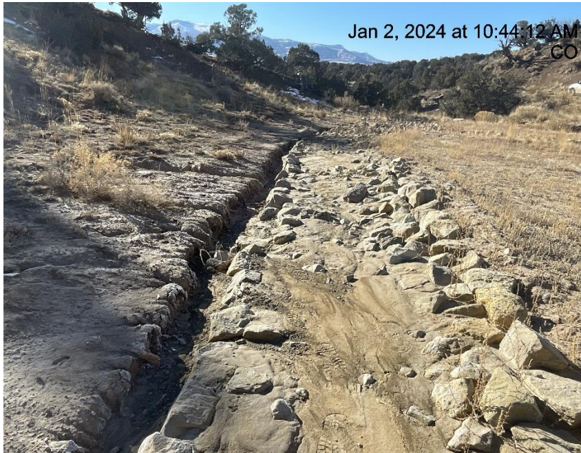
Photo # 1393 Rip Rap Run needs maintenance (eastern side of location)
