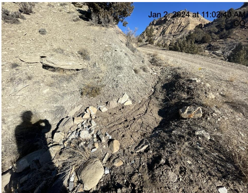
Photo # 1399 Stormwater BMP's along lease road need maintenance (Approximately 75-80 yards from entrance to location)
