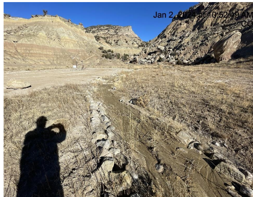
Photo # 1400 Rip Rap Run/BMP needs maintenance (S/SE area of location)
