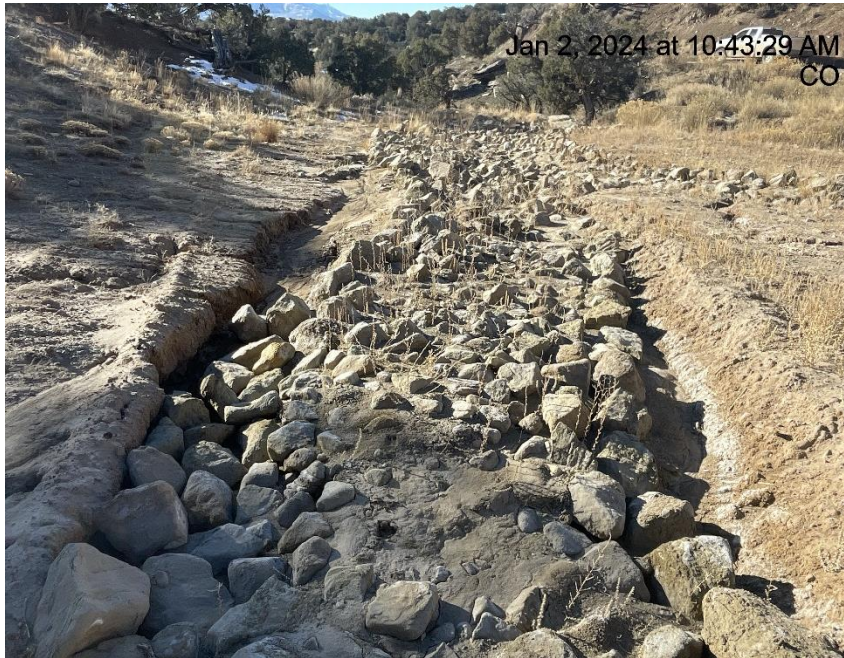
Photo # 1391 Rip Rap Run needs maintenance, stormwater has eroded around both sides of BMP (eastern side of location)
