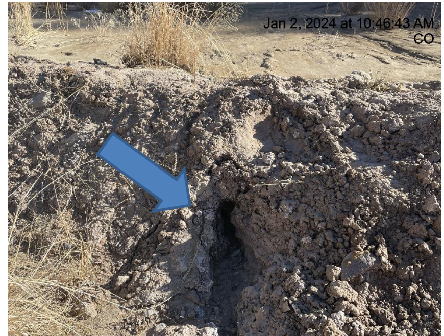
Photo # 1394 Berm needs maintenance/tunnel erosion & transport of sediment through berm & onto location (North area of location)
