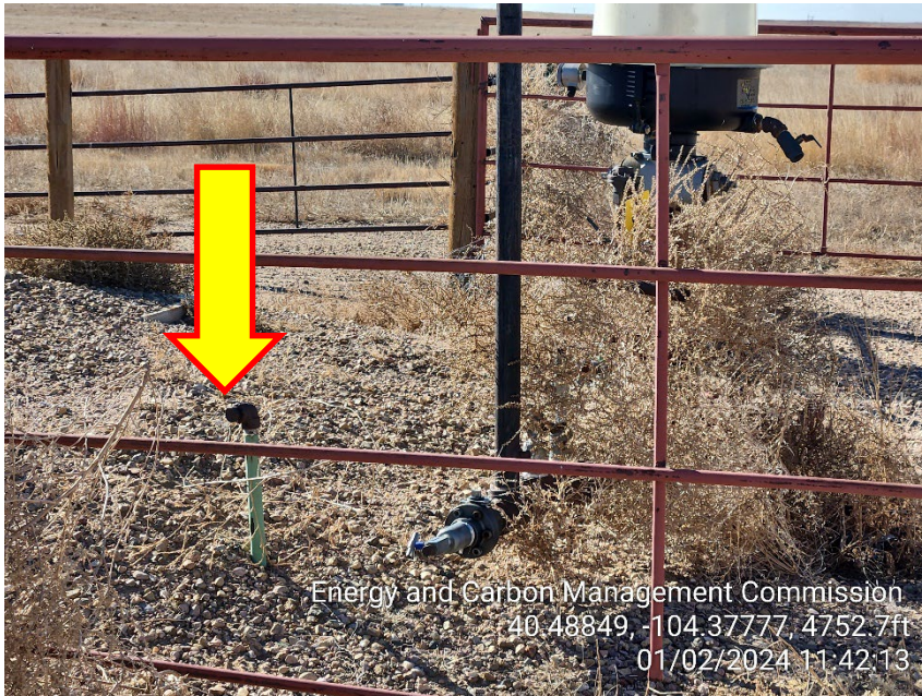
Photo 7 – 1" Unmarked Riser
