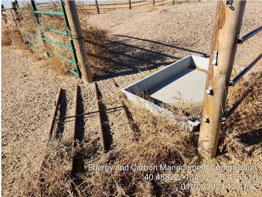
Photo 5 – Unused Secondary Containment
