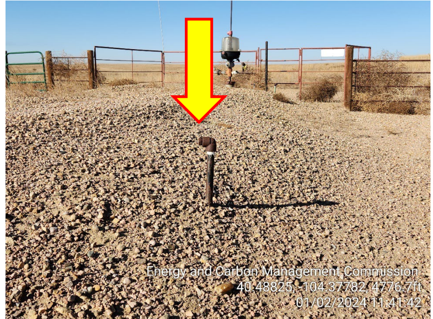
Photo 6 – 1" Unmarked Risers
