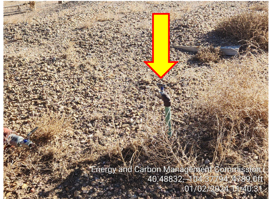
Photo 2 – 1" Unmarked Riser
