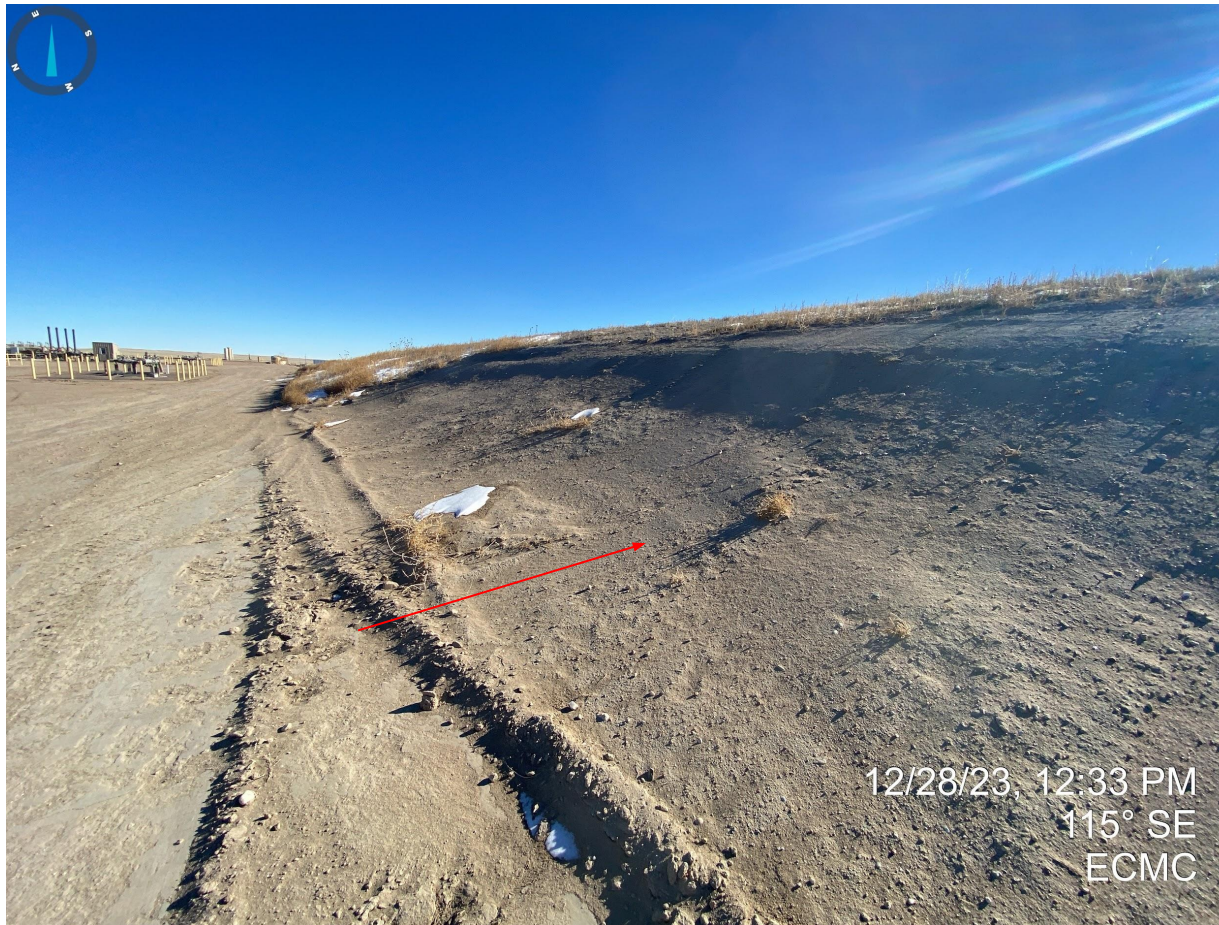
Photo 11. Bare and exposed cuts banks along the southern portion of the production facility are not properly stabilized against wind and water erosion degradation. Additional stabilization measures/BMPs are required.
