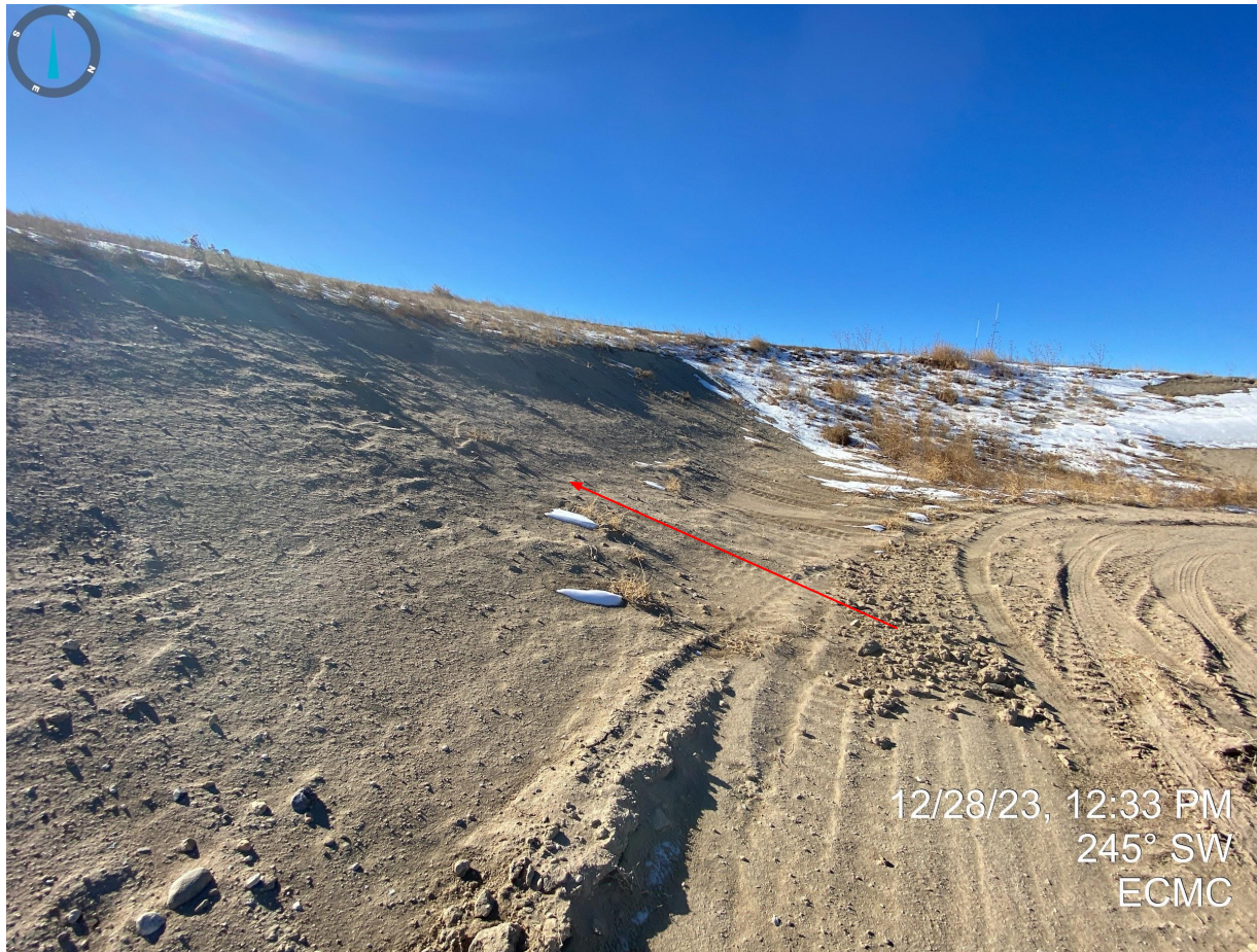
Photo 12. Bare and exposed cuts banks along the southern/southwestern portion of the production facility are not properly stabilized against wind and water erosion degradation. Additional stabilization measures/BMPs are required.
