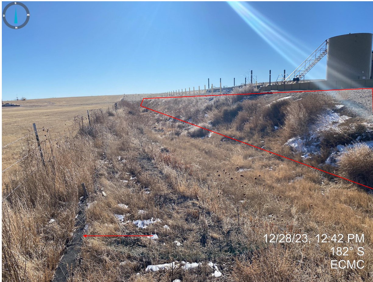
Photo 19. Weedy debris observed around the eastern portion of the production areas. Also pictured, buried/degraded straw wattles that are now considered debris.
