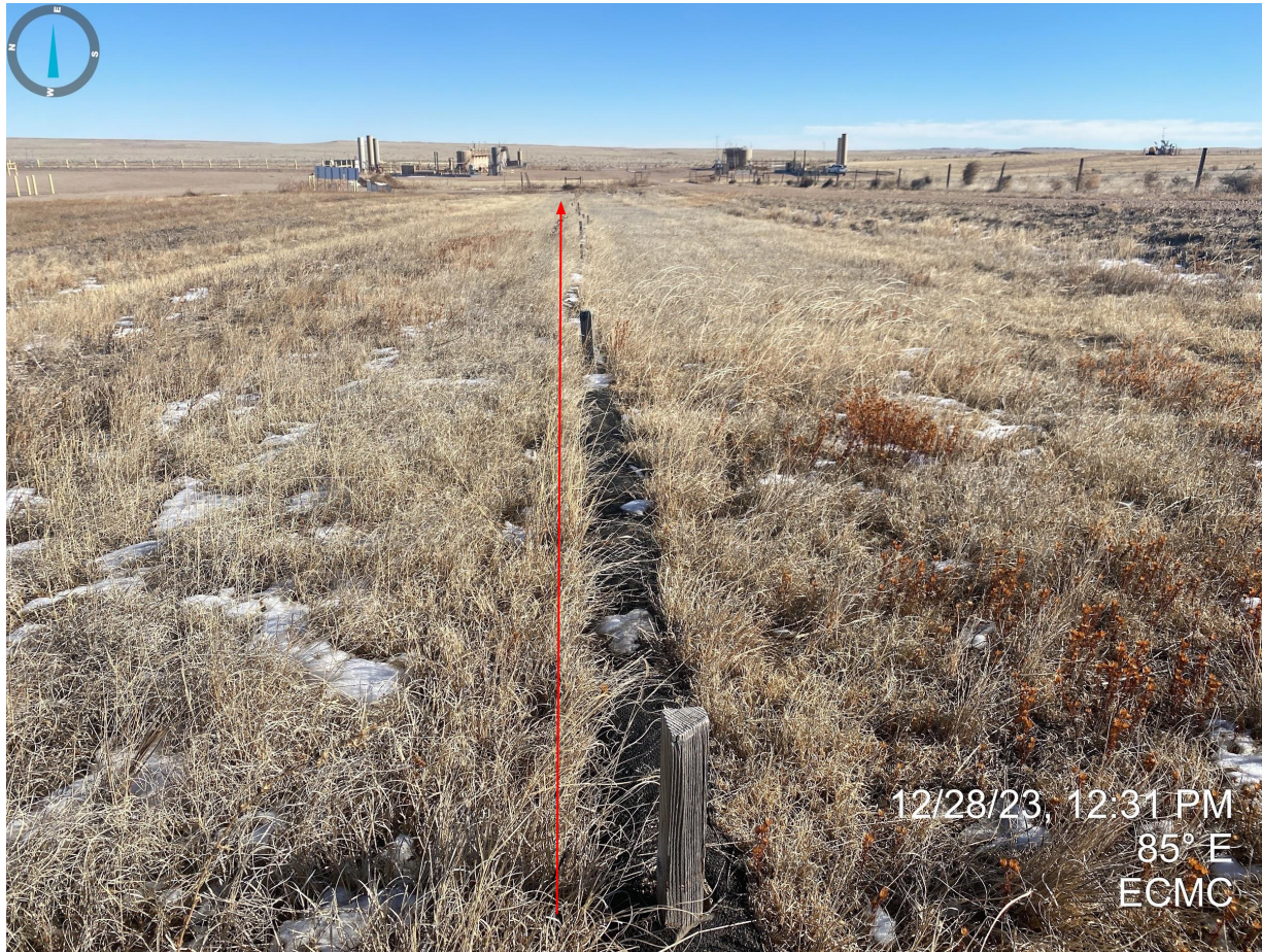
Photo 9. Buried/degraded straw wattles located within the southern interim areas, south of the production facility, are now considered debris as they are no longer a properly functioning control measure/BMP.
