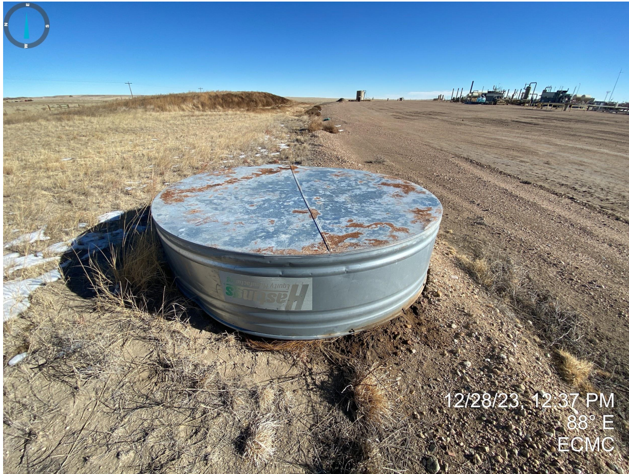
Photo 15. Stock tank/secondary containment does not appear to be in use and needs to be removed or returned to service.
