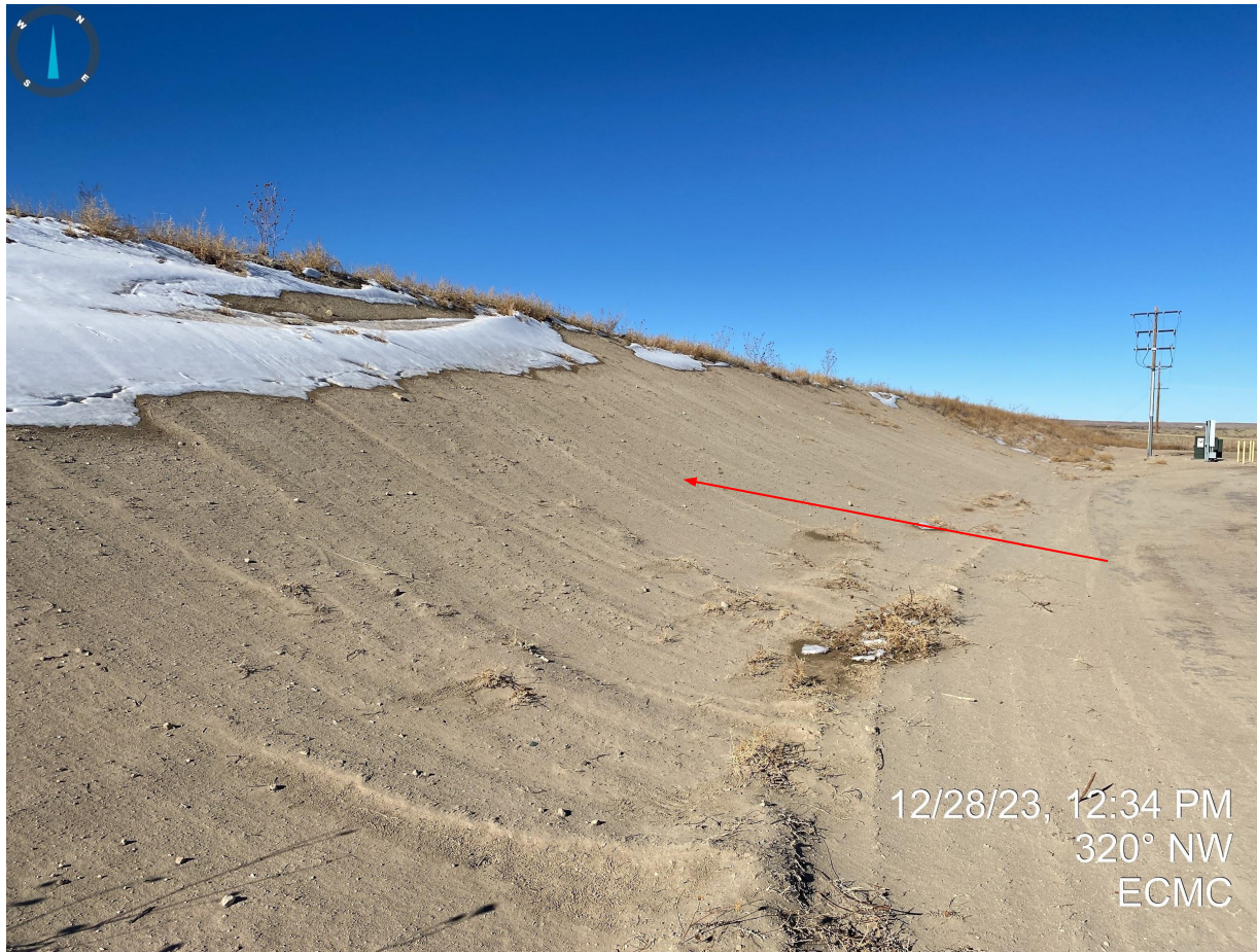
Photo 13. Bare and exposed cuts banks along the western/southwestern portion of the production facility are not properly stabilized against wind and water erosion degradation. Additional stabilization measures/BMPs are required.
