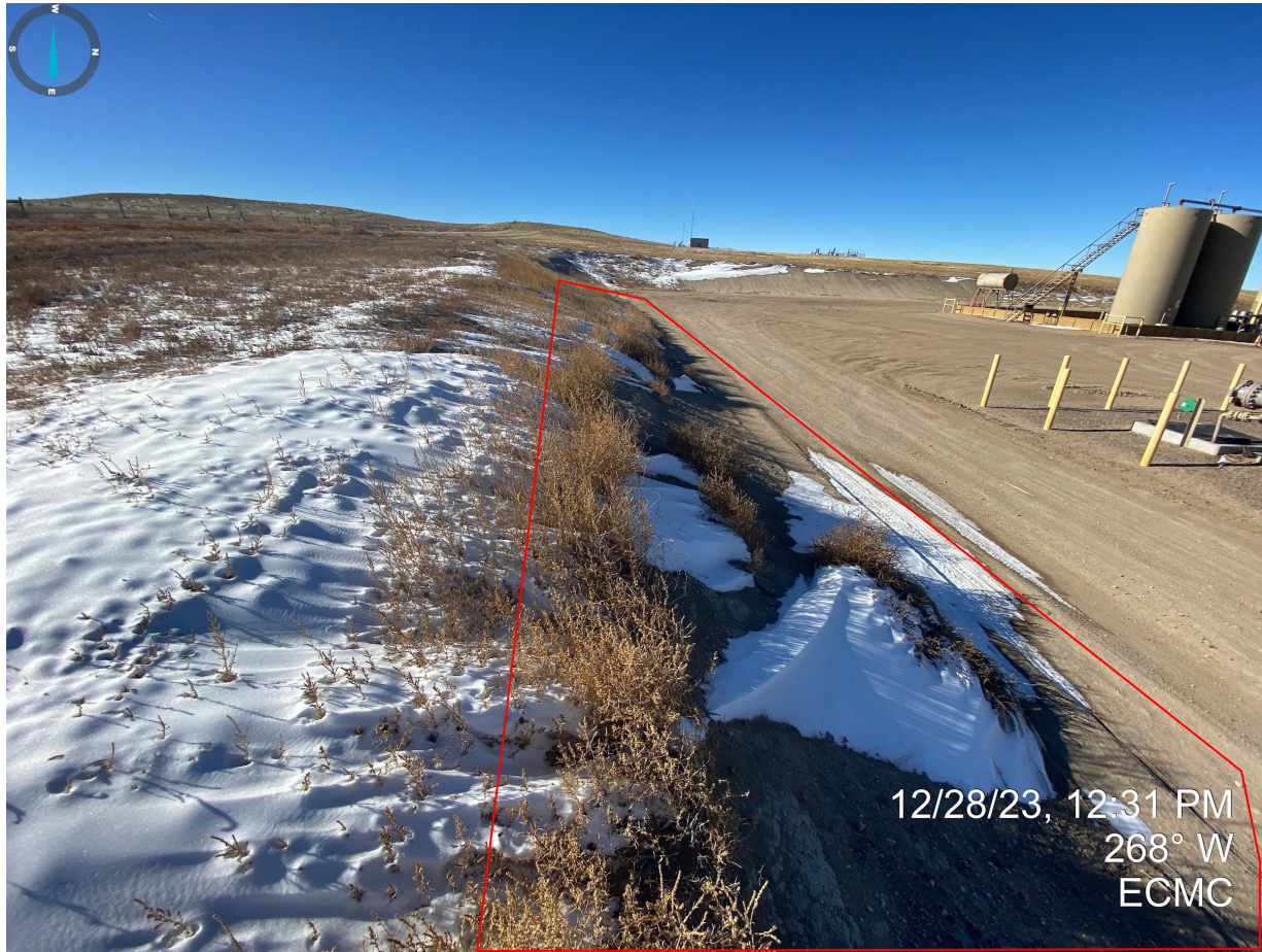
Photo 10. Weedy debris and bare/exposed cut banks along the southern portion of the production areas.
