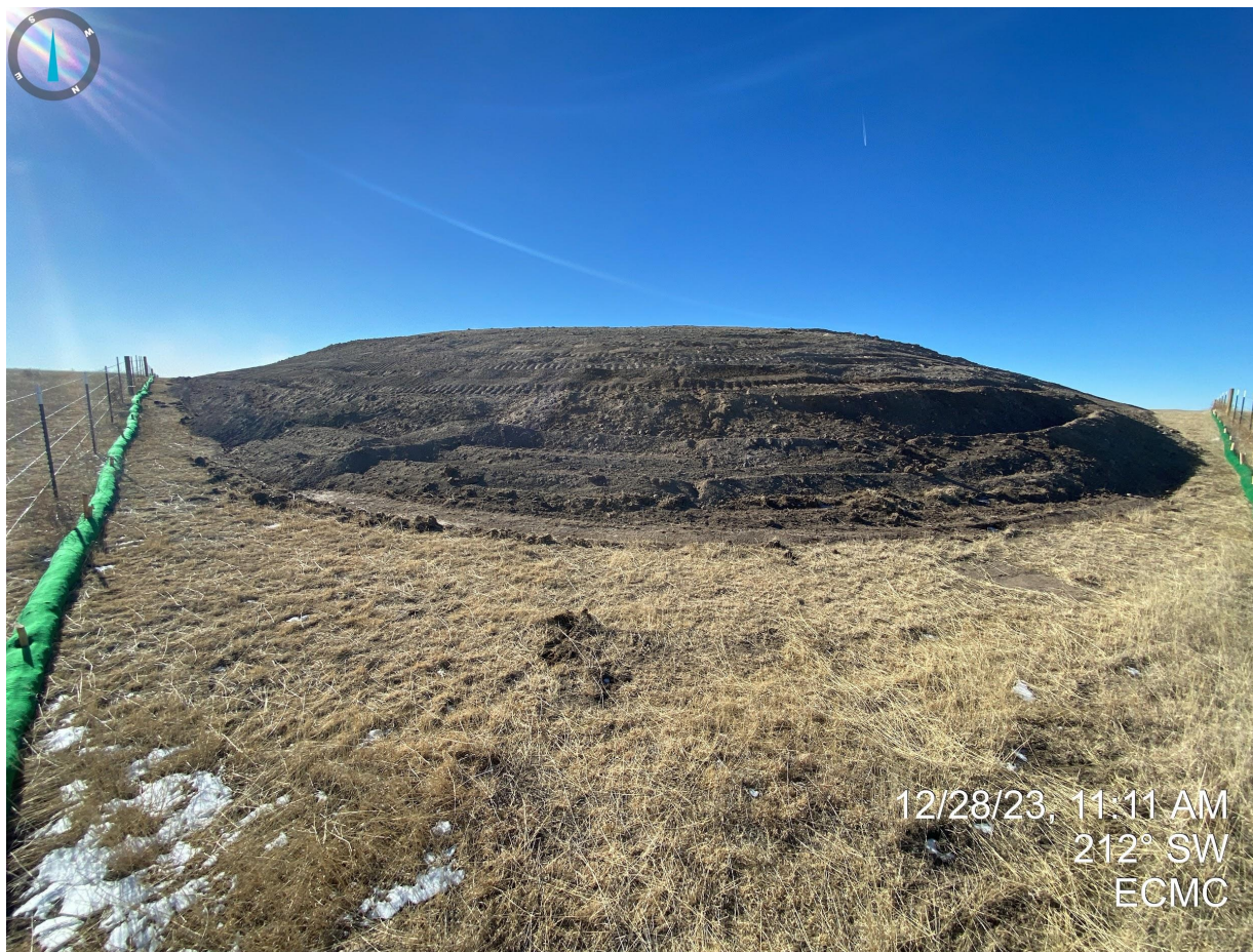
Photo 25. Taken from the northeast corner; facing the topsoil stockpile. Topsoil salvage operations were still ongoing at the time of this inspection; the Operator shall ensure that all stockpile soils are stabilized per Rule 1002.c.
