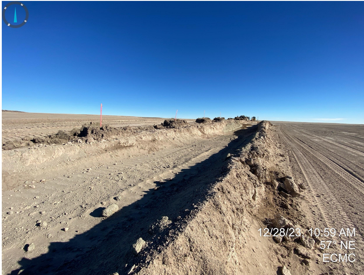
Photo 9. Taken from the center portion of the location; facing northeast. Photo illustrates cut and fill activities occurring near the proposed well locations.
