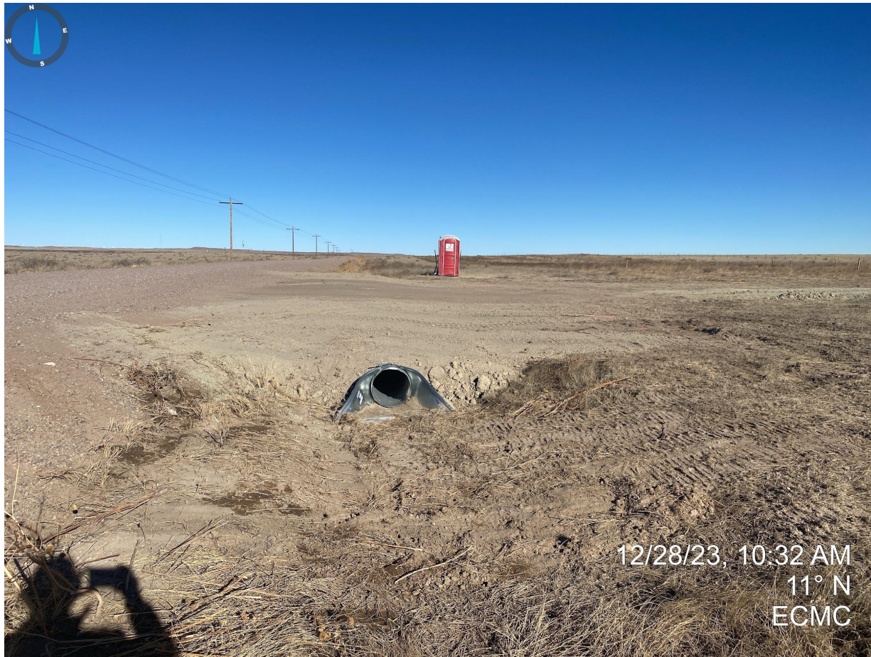
Photo 2. Taken from the county road near the location entrance. A culvert has been installed in the bar ditch.
