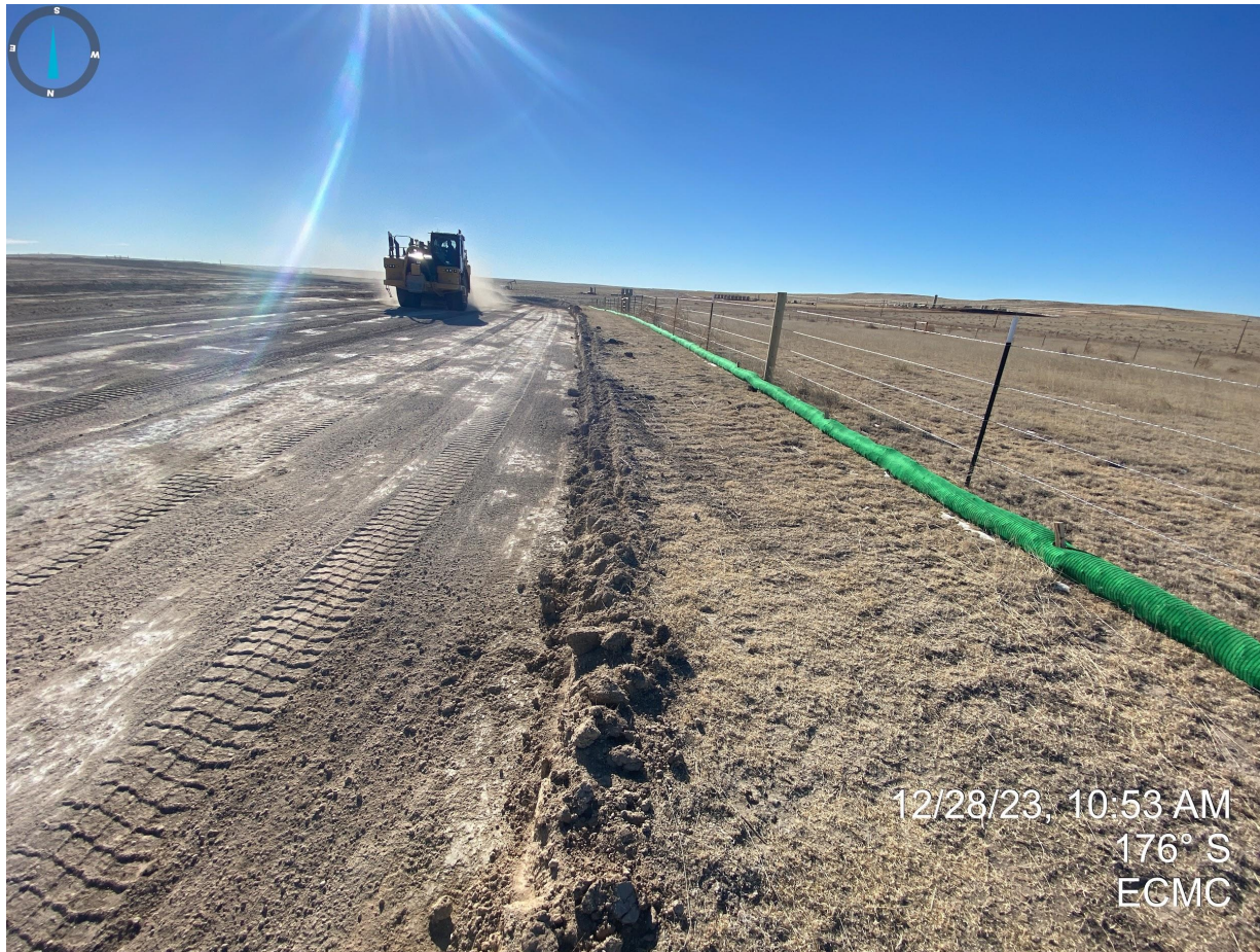
Photo 5. West side of location. Photo illustrates topsoil salvage activities are still ongoing at the time of this inspection.
