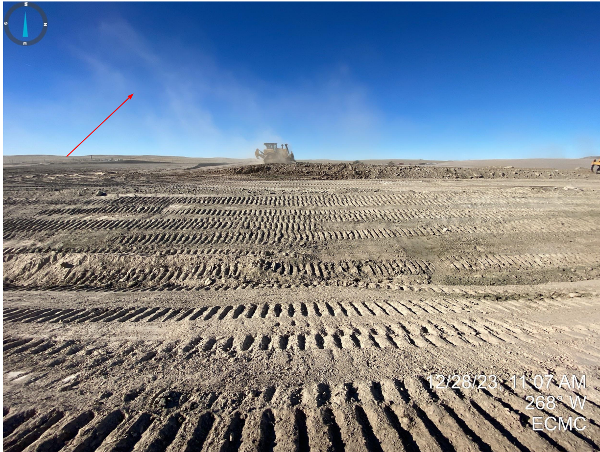
Photo 19. Photo illustrates fugitive dust occurring from dirt work activities. There were no dust suppression BMPs observed during this inspection.
