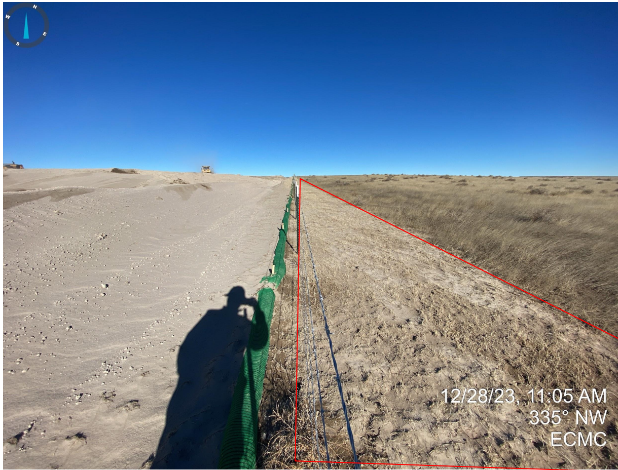
Photo 15. Taken from the southeast corner, facing northwest. Photo illustrates blow sand originating from the unstabilized soils of the construction area.
