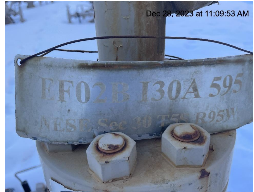
Photo # 1071 Wellhead signs lack required information
