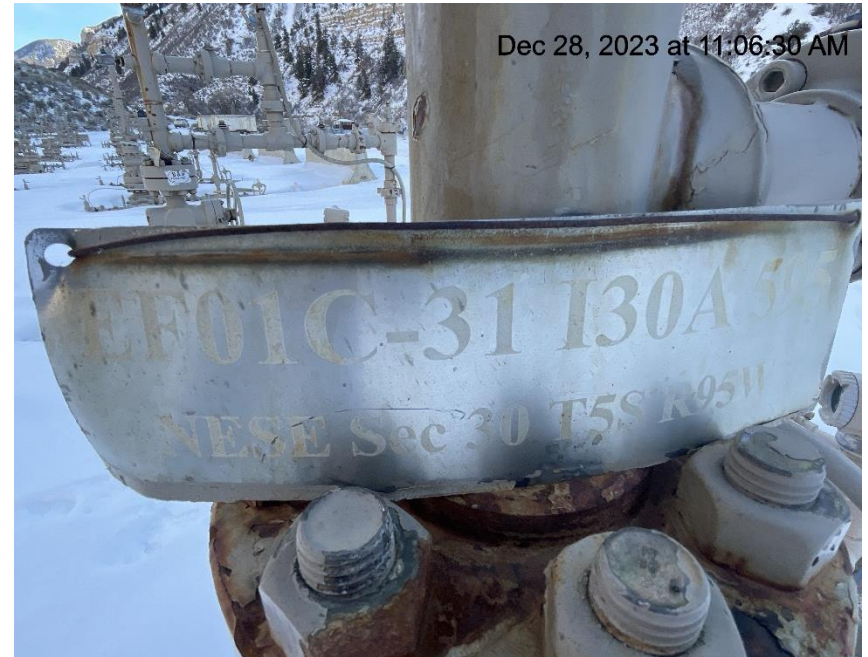
Photo # 1067 Wellhead signs lack required information
