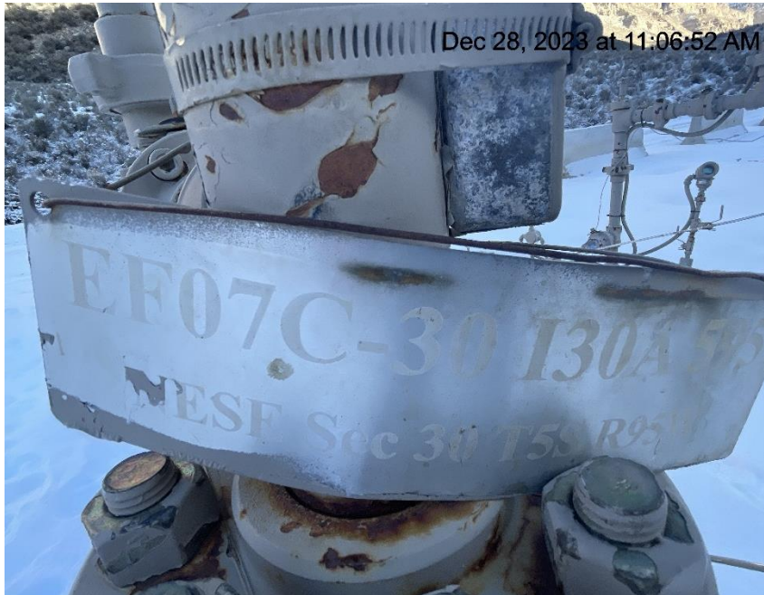
Photo # 1068 Wellhead signs lack required information
