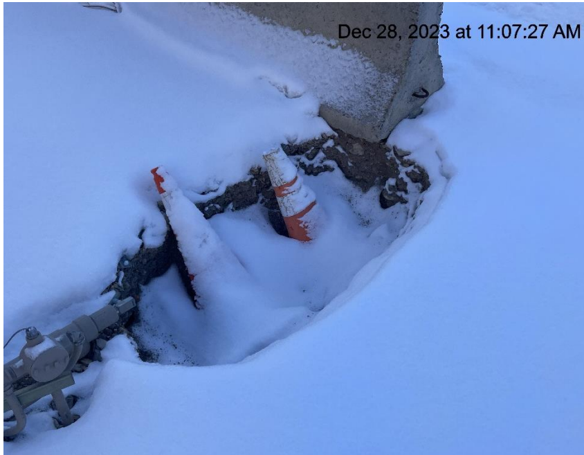
Photo # 1066 Hole in ground near wellheads/wildlife & personnel protection insufficient
