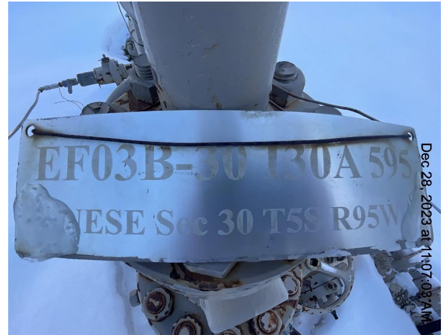
Photo # 1069 Wellhead signs lack required information
