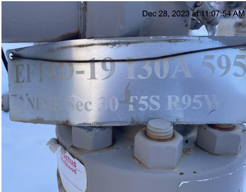
Photo # 1070 Wellhead signs lack required information
