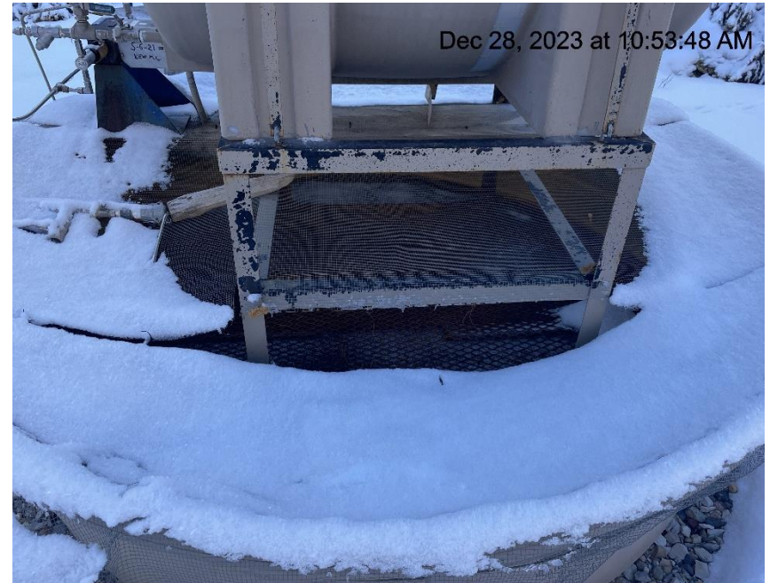
Photo # 1075 Wildlife protection on chemical tank containment needs maintenance
