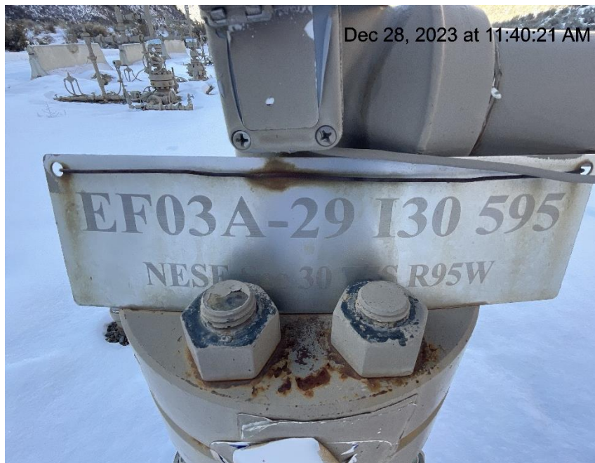
Photo # 1116 Wellhead signs lack required information
