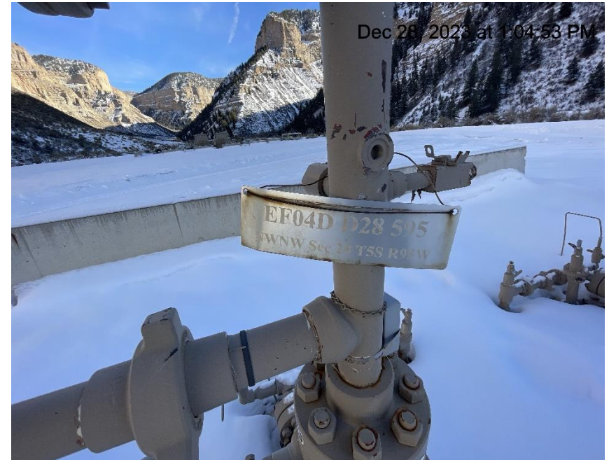
Photo # 1260 Wellhead signs lack required information
