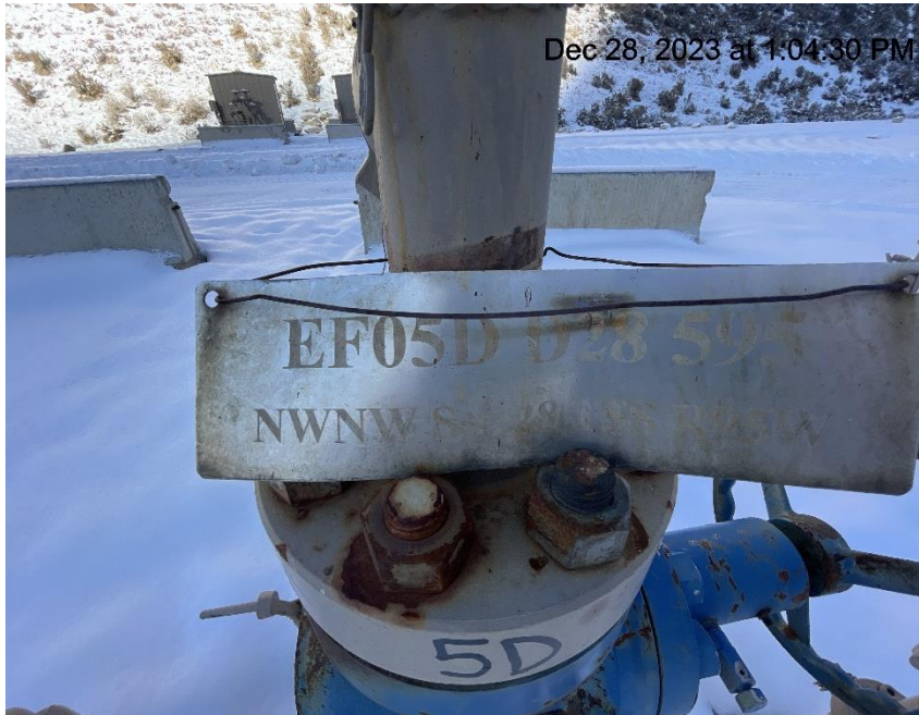
Photo # 1259 Wellhead signs lack required information
