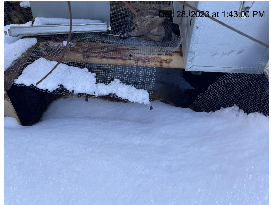
Photo # 1329 Wildlife protection on chemical tank containment needs maintenance
