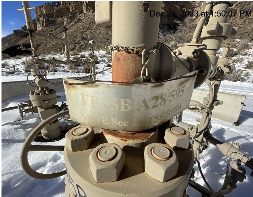
Photo # 1328 Wellhead sign lacks required info
