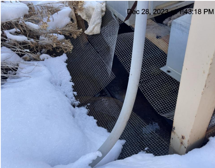
Photo # 1330 Wildlife protection on chemical tank containment needs maintenance
