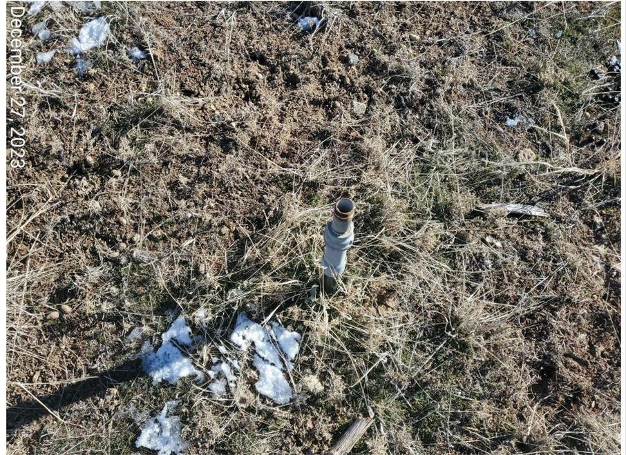
**Photo 6:** Photo show uncapped riser on the southeastern interim areas of the Location. Riser is considered unused equipment and requires removal.
