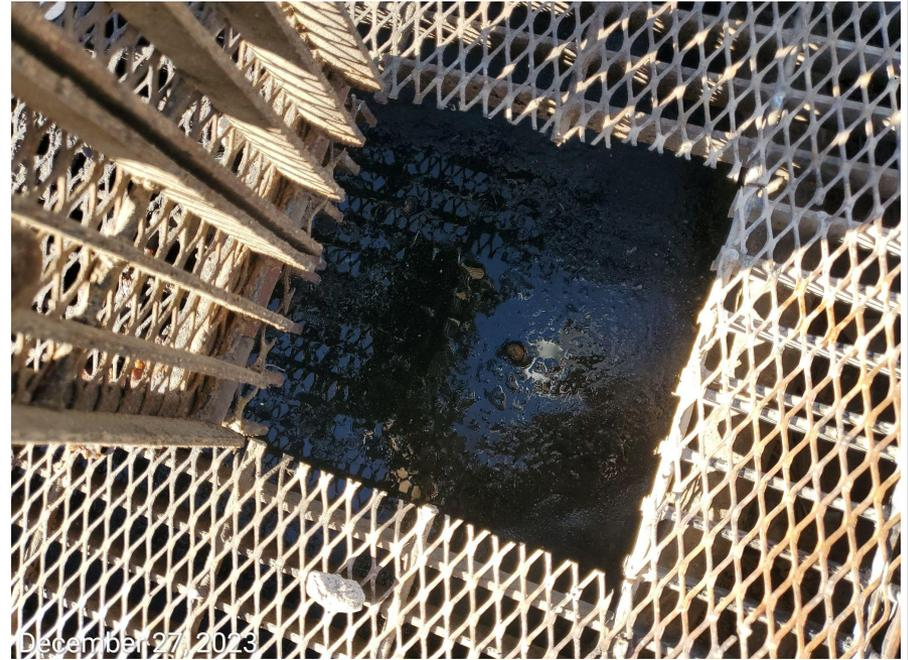
**Photo 3:** Photo taken from the pipeline equipment on the west end of the Location. Leak evident at equipment. Photo right shows fluids spilled into containment.
