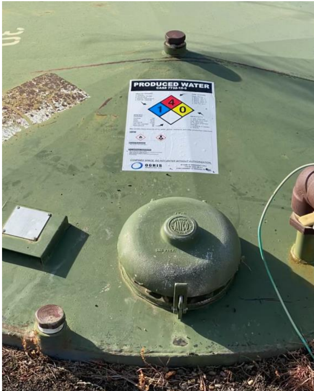
PHOTO 3: THE HATCH DOOR ON THE PRODUCED WATER TANK HAS BEEN CLOSED AND LATCHED. THE SELF INSPECTION PROCESS HAS BEEN REVIEWED.
