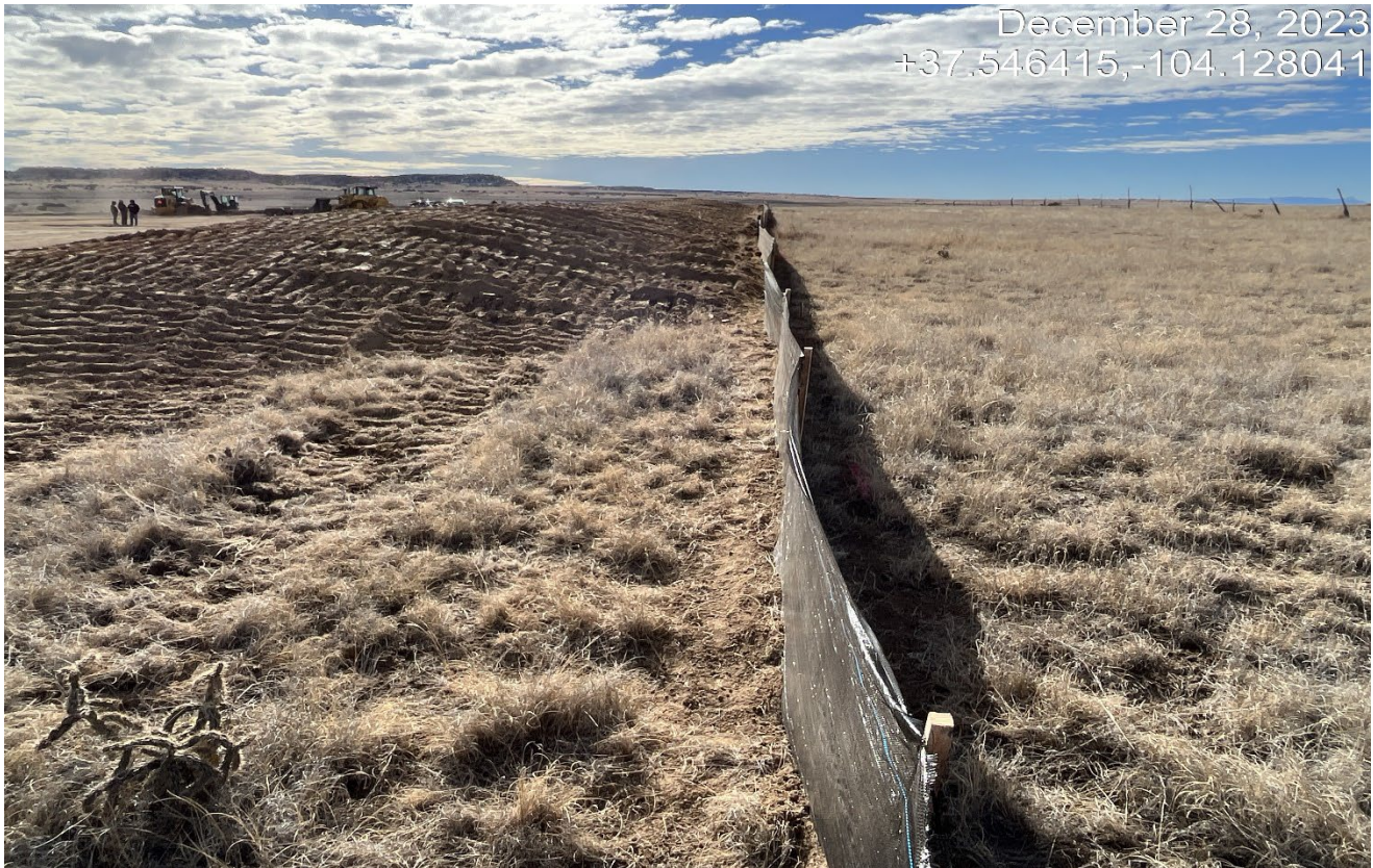
Photo 5. Facing southeast. There is a perimeter silt fence installed around the location.
