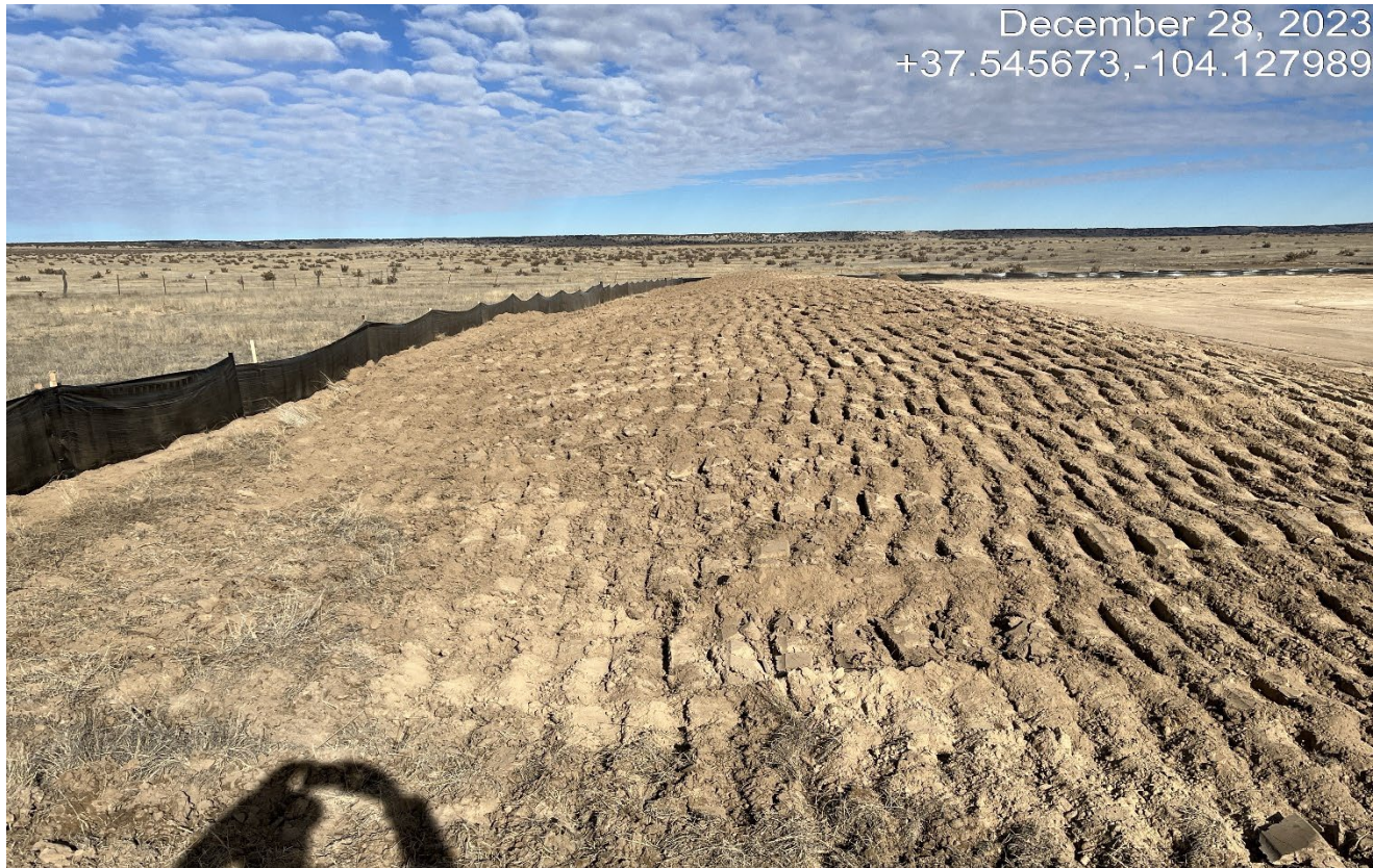
Photo 3. There is a topsoil pile stored and stabilized at the west side of the location. Approximately 270' x 20'.
