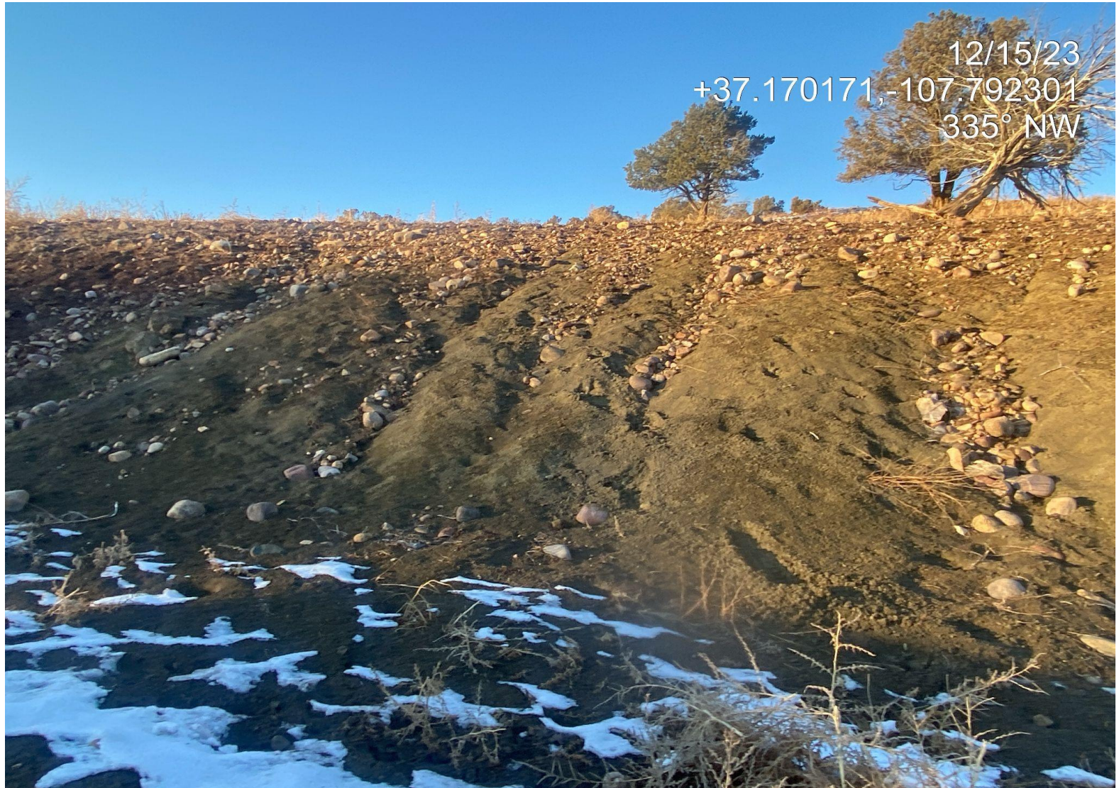
Photo 2. View of rill erosion observed forming on the northern fill slope interim area which also lacks vegetation needed for stabilization.
