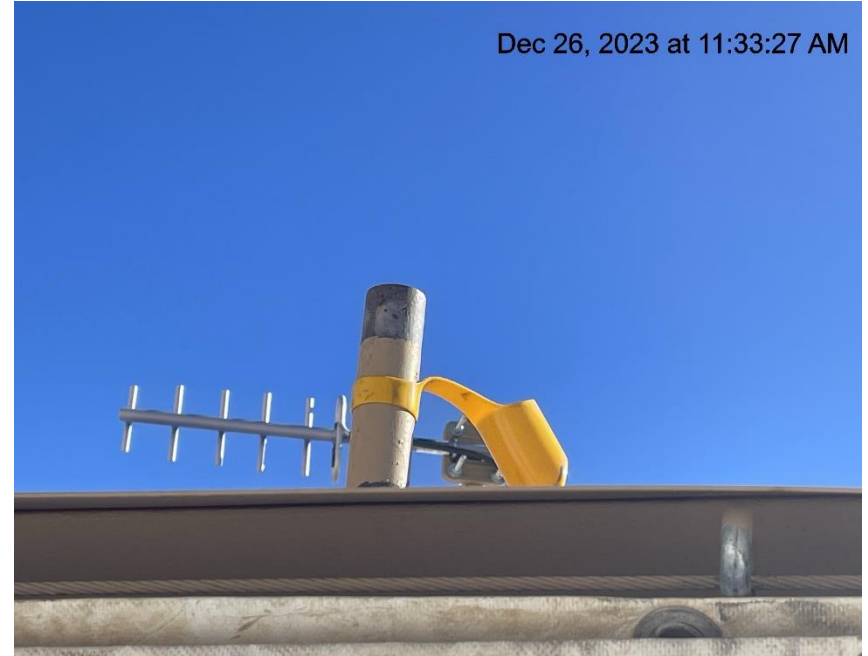
Photo # 758 Cap not covering PRV vent line on test separator
