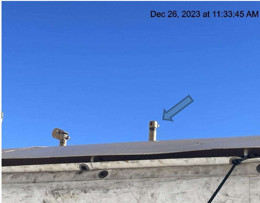
Photo # 759 PRV vent line on test separator lacks cap
