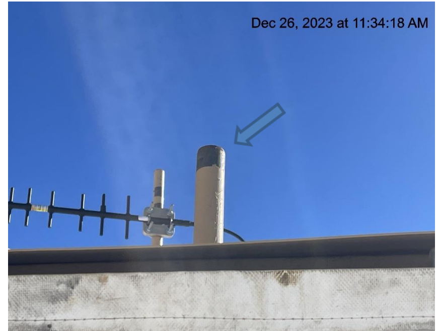
Photo # 760 PRV vent line on test separator lacks cap
