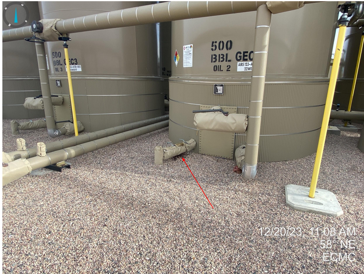
Photo 1. Stained soil observed near tank battery connections.
