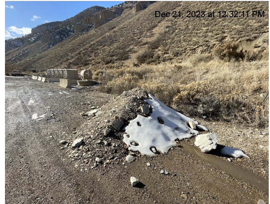
Photo # 630 Stockpiled soils with no BMP's
