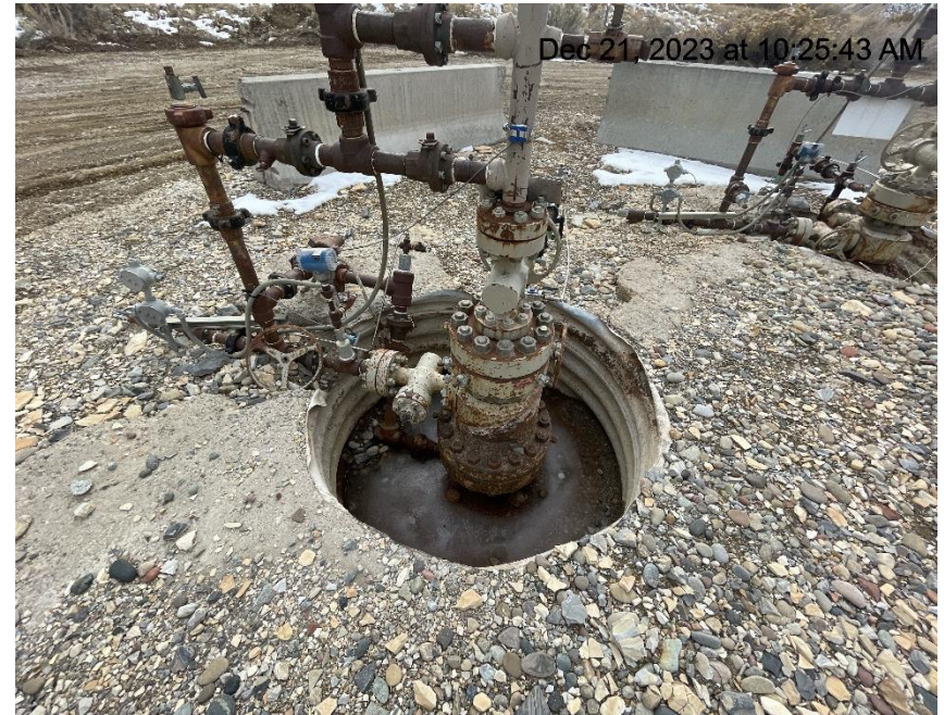
Photo # 429 Open wellhead cellar
