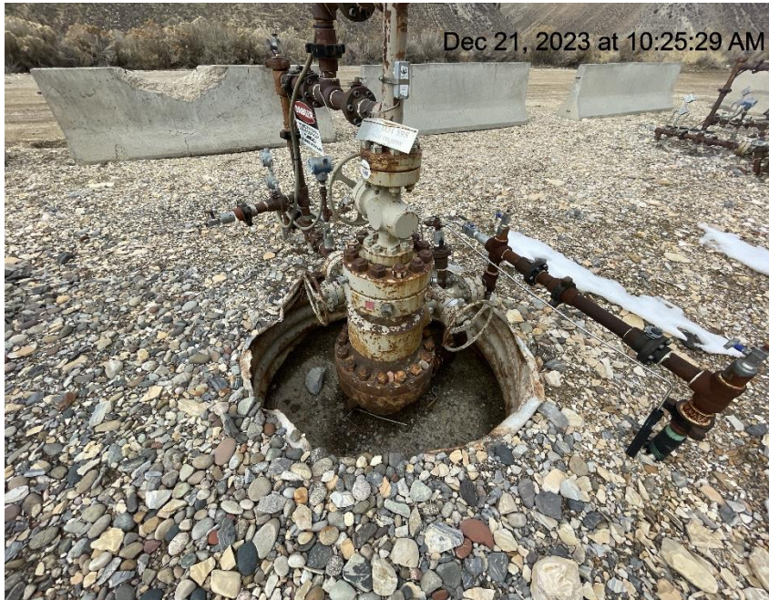
Photo # 428 Open wellhead cellar
