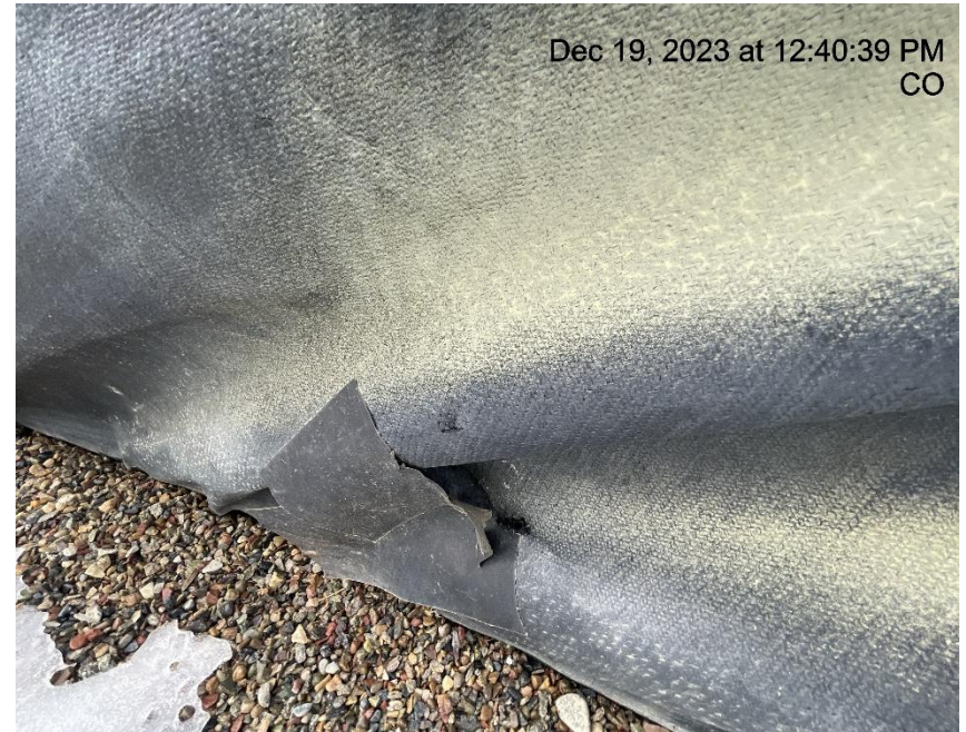
Photo # 308 Hole in liner/liner needs maintenance
