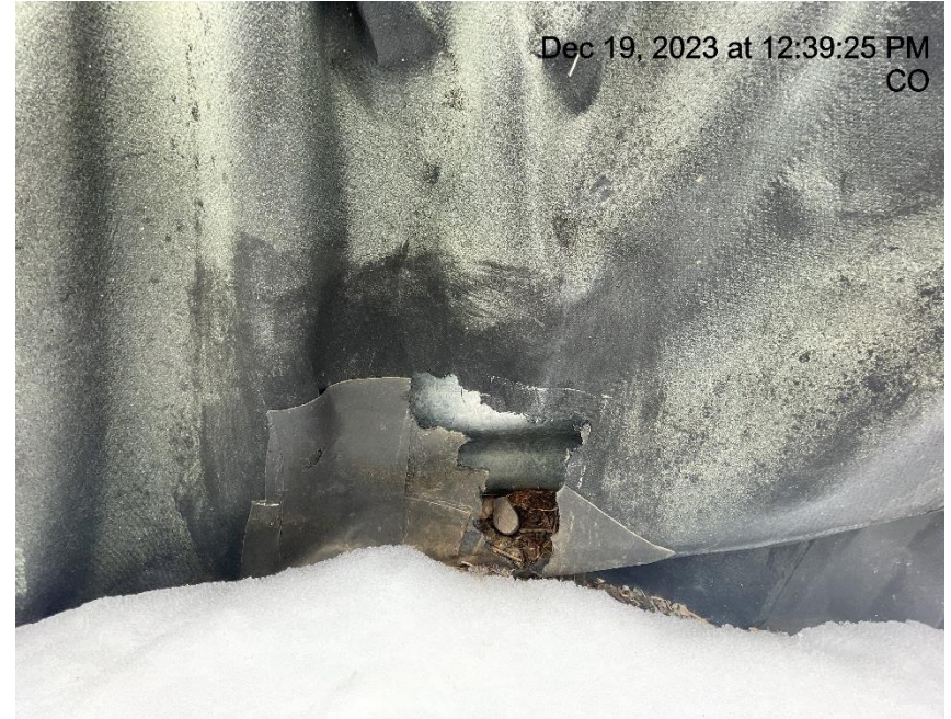
Photo # 298 Hole in liner/liner needs maintenance
