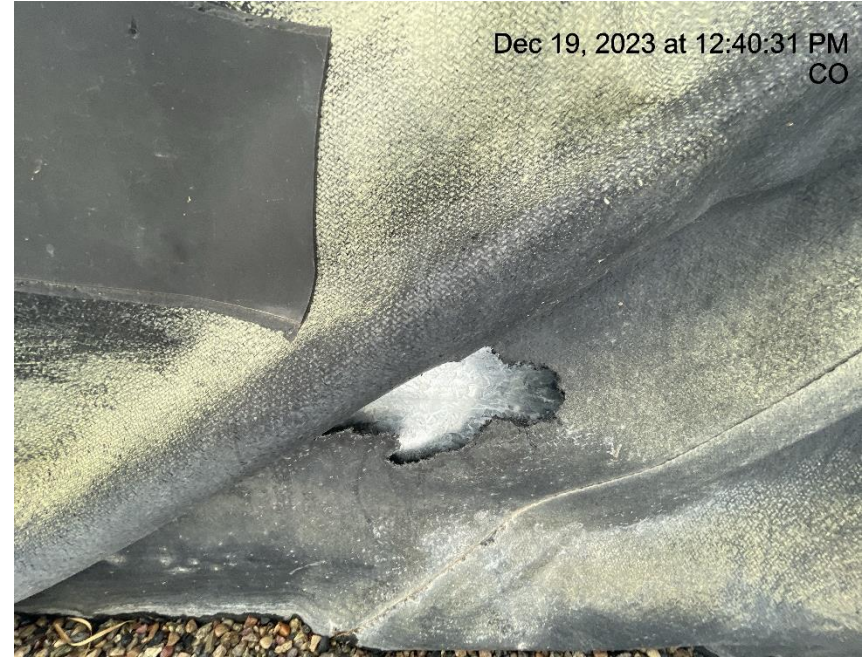
Photo # 306 Hole in liner/liner needs maintenance
