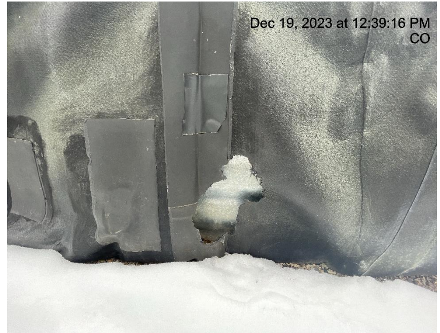
Photo # 296 Hole in liner/liner needs maintenance
