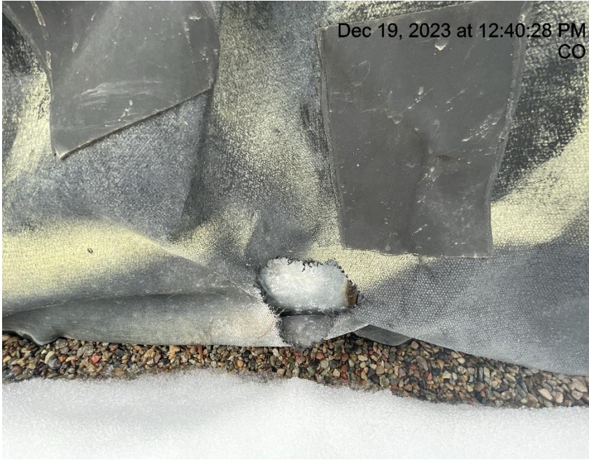
Photo # 305 Hole in liner/liner needs maintenance
