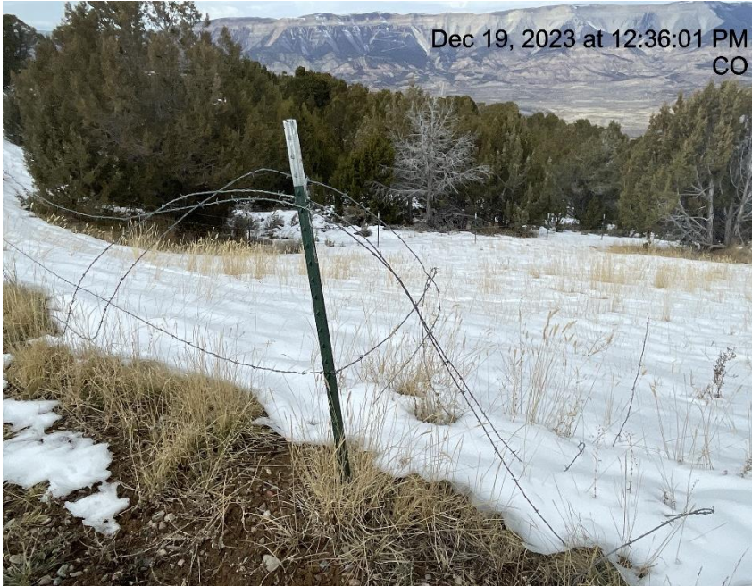
Photo # 293 Barbed wire fence needs maintenance/wildlife hazard
