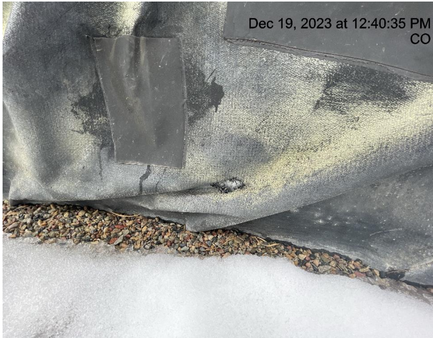
Photo # 307 Hole in liner/liner needs maintenance
