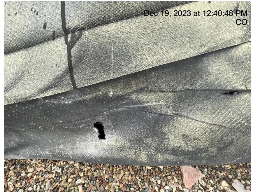
Photo # 310 Hole in liner/liner needs maintenance
