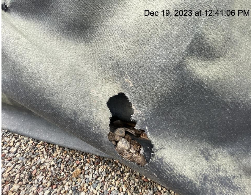
Photo # 314 Hole in liner/liner needs maintenance
