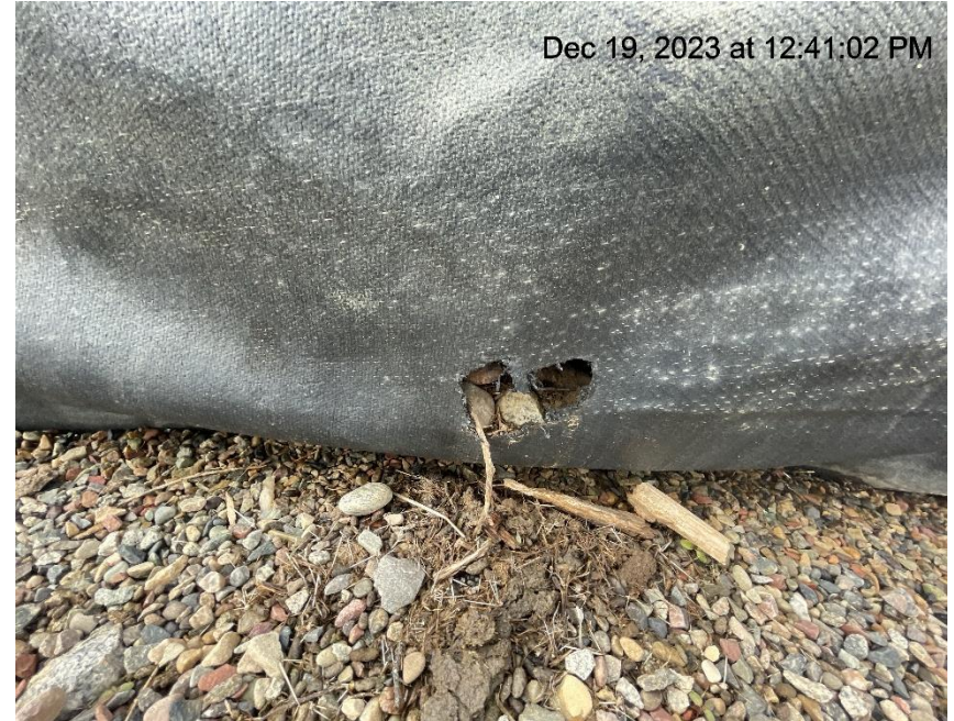
Photo # 312 Hole in liner/liner needs maintenance
