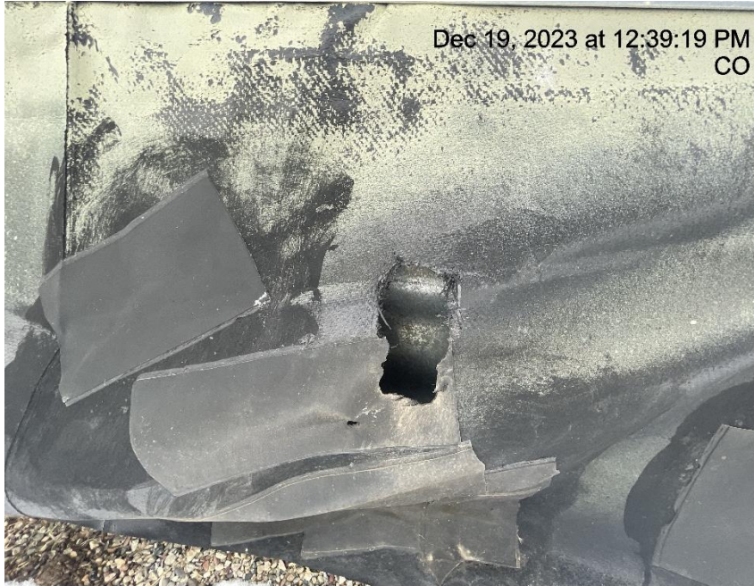
Photo # 297 Hole in liner/liner needs maintenance
