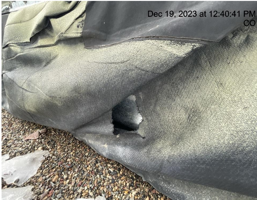
Photo # 309 Hole in liner/liner needs maintenance
