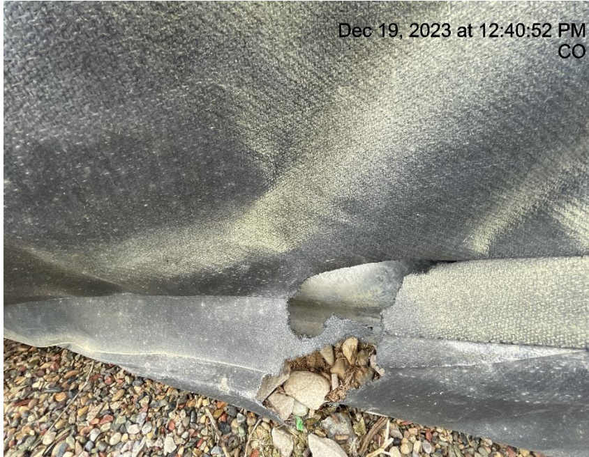
Photo # 311 Hole in liner/liner needs maintenance
