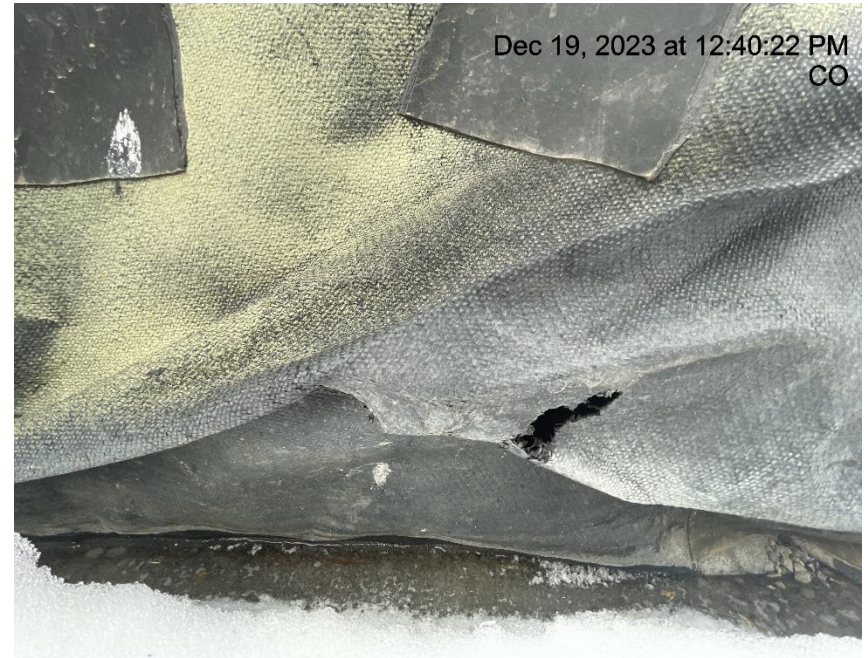
Photo # 304 Hole in liner/liner needs maintenance
