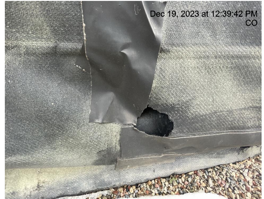
Photo # 300 Hole in liner/liner needs maintenance
