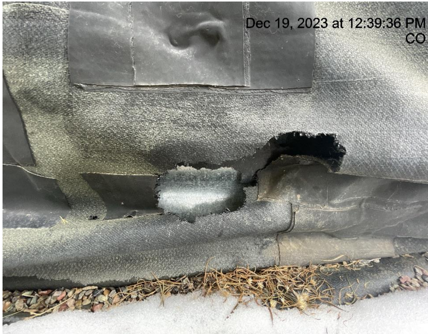
Photo # 299 Hole in liner/liner needs maintenance
