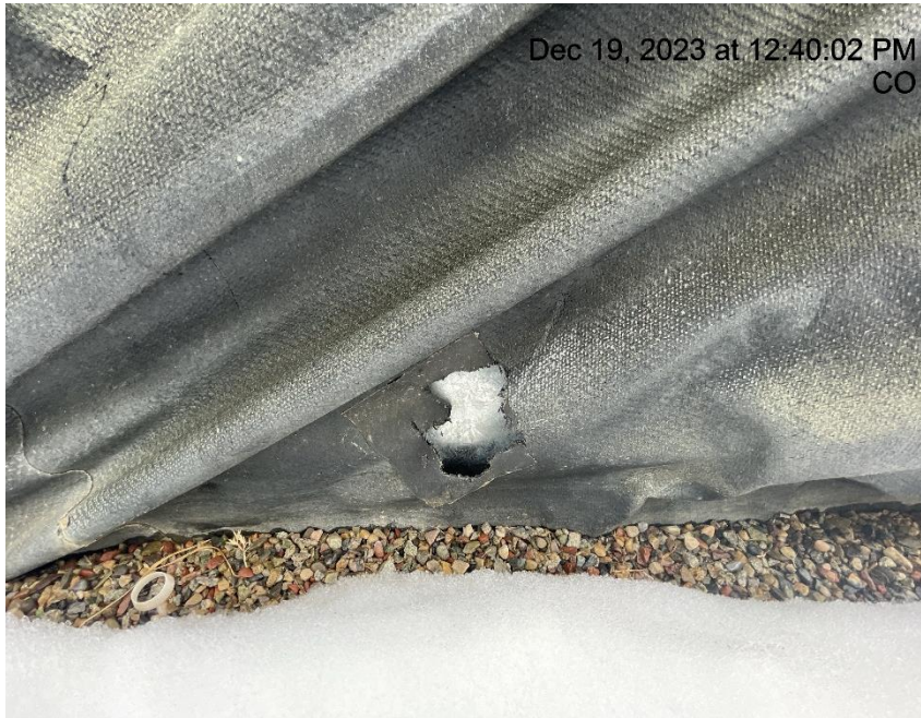
Photo # 301 Hole in liner/liner needs maintenance
