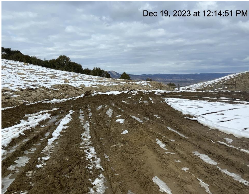
Photo # 222 Lack of stabilization/compaction/insufficient BMP's
