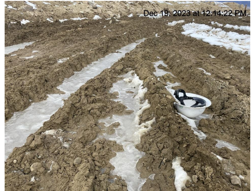
Photo # 219 Lack of stabilization/compaction/insufficient BMP's
