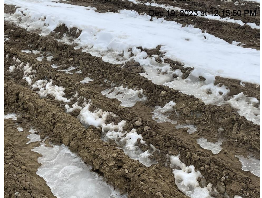
Photo # 225 Lack of stabilization/compaction/insufficient BMP's
