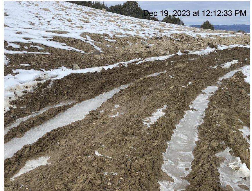
Photo # 215 Lack of stabilization/compaction/insufficient BMP's
