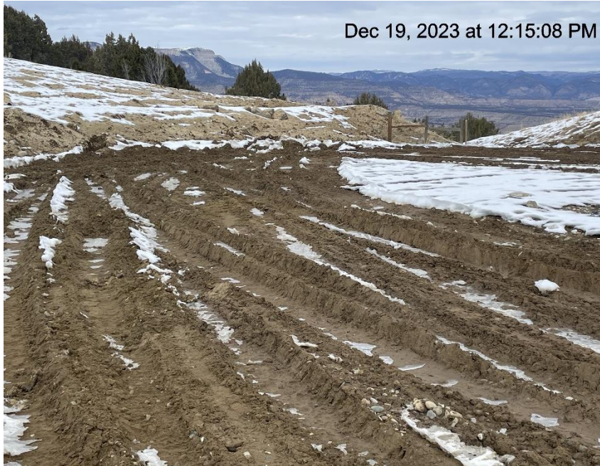
Photo # 224 Lack of stabilization/compaction/insufficient BMP's
