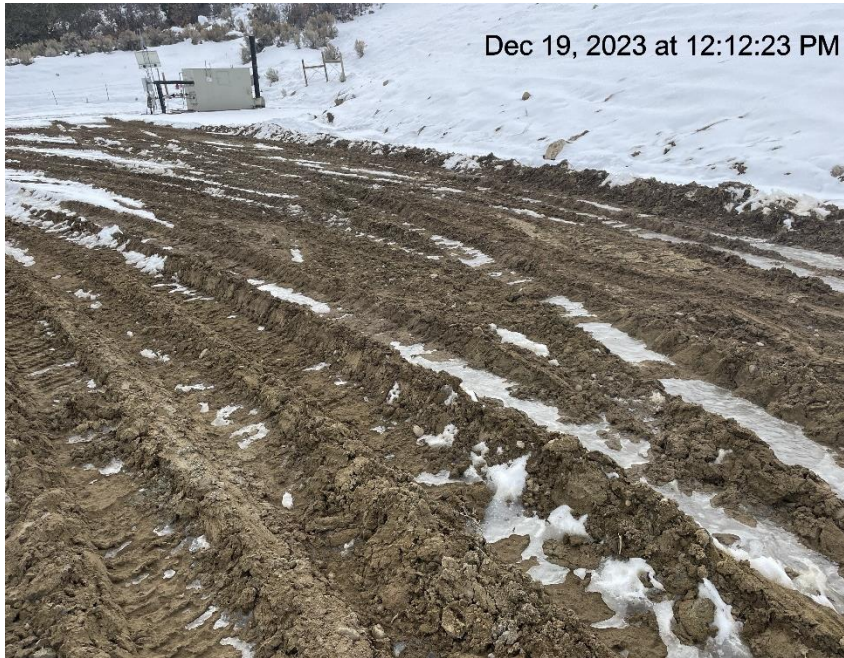
Photo # 214 Lack of stabilization/compaction/insufficient BMP's
