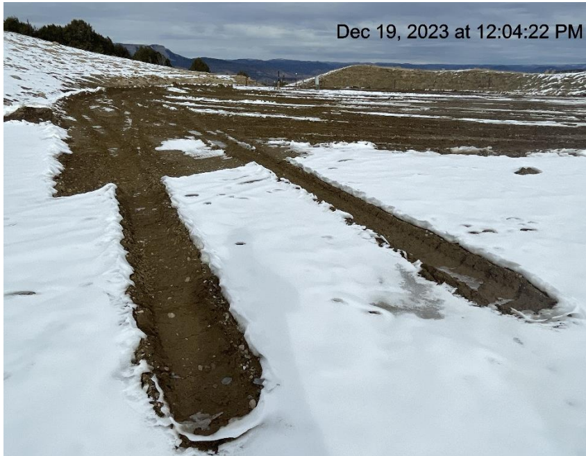
Photo # 200 Lack of stabilization/compaction/ insufficient BMP's
