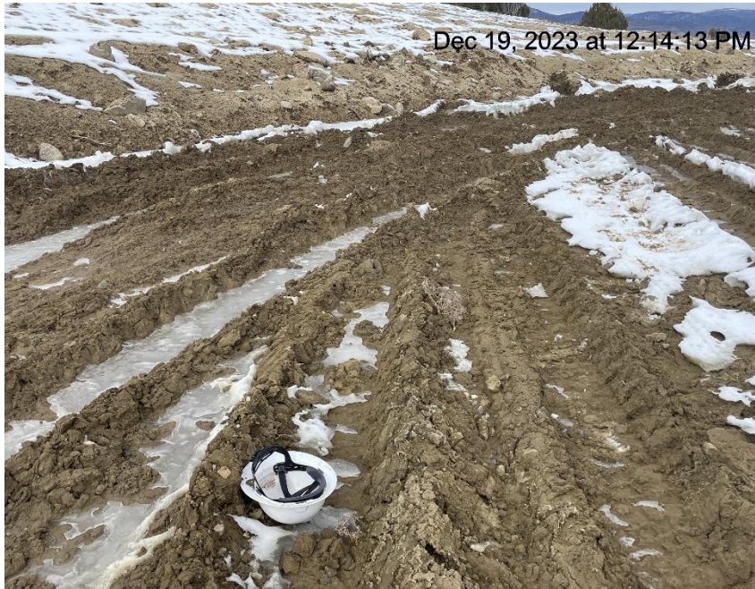
Photo # 218 Lack of stabilization/compaction/insufficient BMP's
