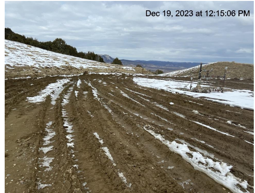
Photo # 223 Lack of stabilization/compaction/insufficient BMP's
