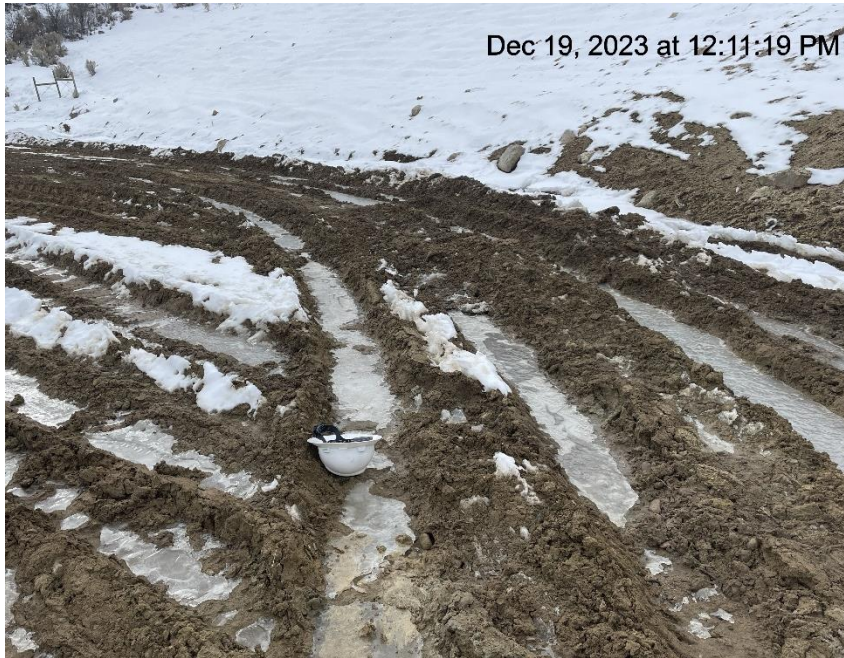
Photo # 208 Lack of stabilization/compaction/insufficient BMP's
