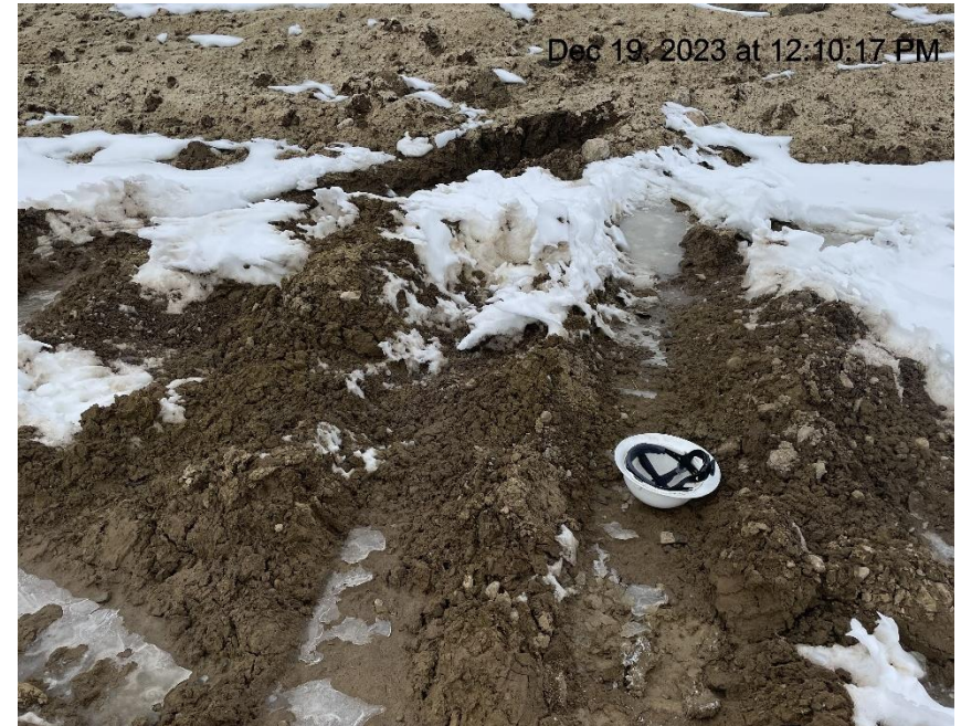
Photo # 203 Lack of stabilization/compaction/insufficient BMP's
