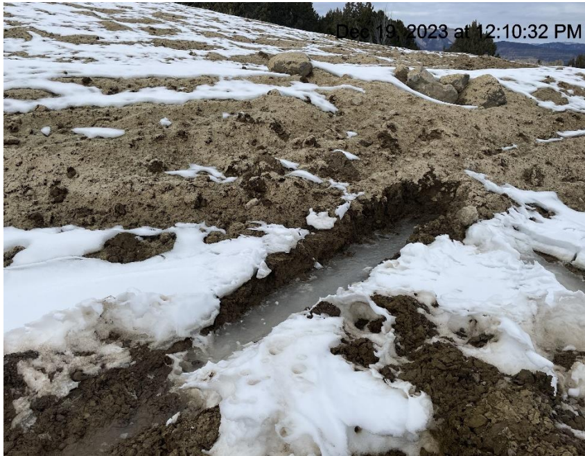
Photo # 204 Lack of stabilization/compaction/insufficient BMP's
