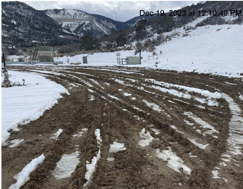
Photo # 206 Lack of stabilization/compaction/insufficient BMP's
