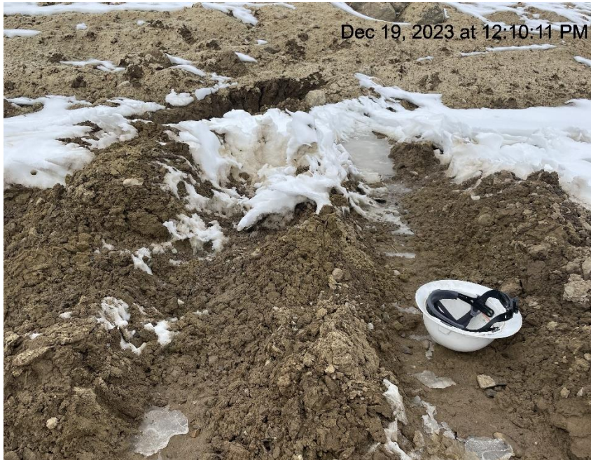
Photo # 202 Lack of stabilization/compaction/insufficient BMP's
