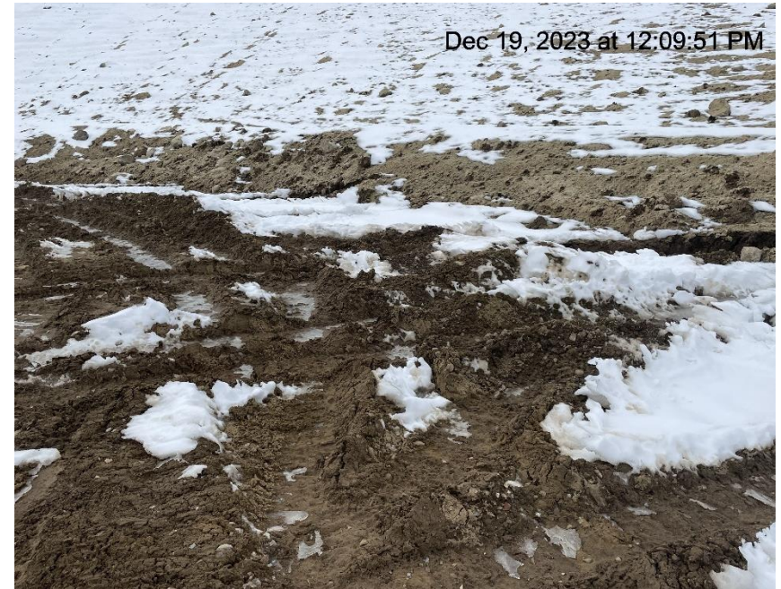
Photo # 201 Lack of stabilization/compaction/insufficient BMP's
