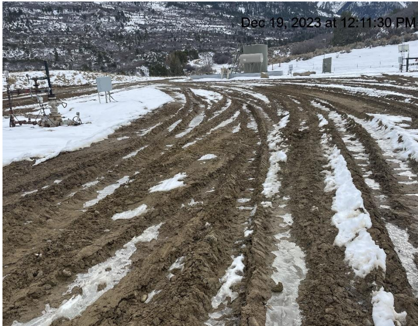
Photo # 210 Lack of stabilization/compaction/insufficient BMP's
