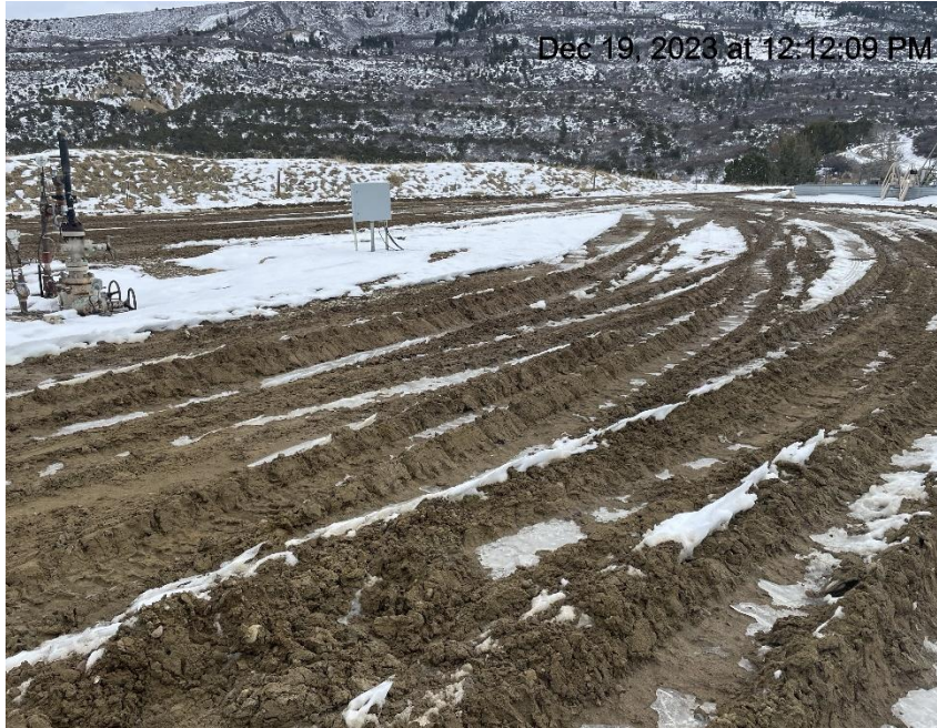
Photo # 212 Lack of stabilization/compaction/insufficient BMP's
