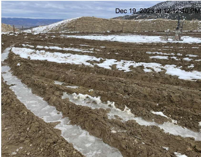
Photo # 216 Lack of stabilization/compaction/insufficient BMP's
