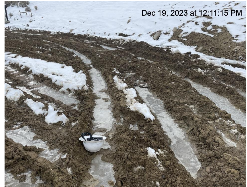
Photo # 207 Lack of stabilization/compaction/insufficient BMP's
