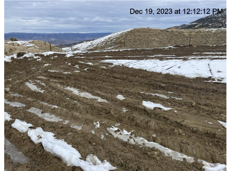
Photo # 213 Lack of stabilization/compaction/insufficient BMP's
