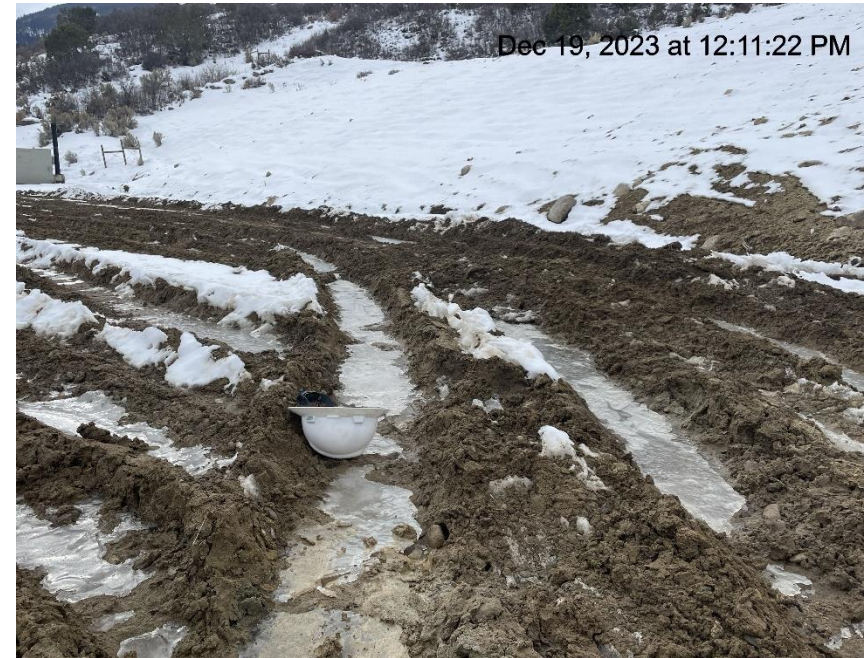
Photo # 209 Lack of stabilization/compaction/insufficient BMP's
