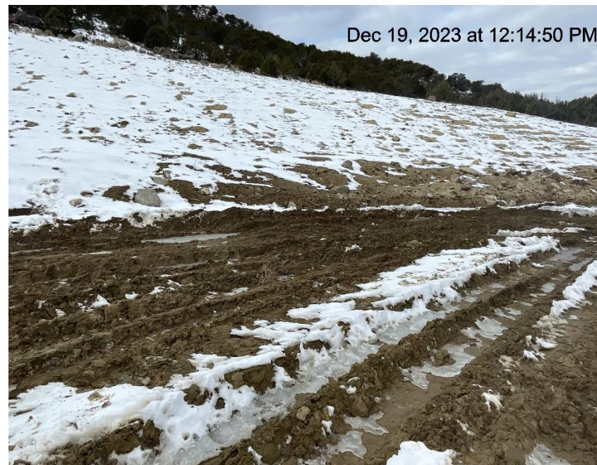
Photo # 221 Lack of stabilization/compaction/insufficient BMP's
