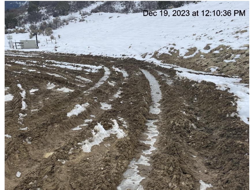
Photo # 205 Lack of stabilization/compaction/insufficient BMP's
