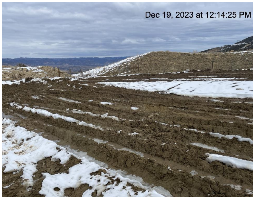
Photo # 220 Lack of stabilization/compaction/insufficient BMP's
