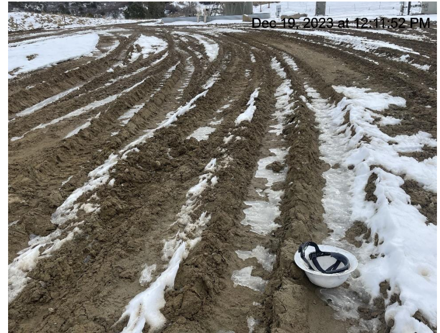
Photo # 211 Lack of stabilization/compaction/insufficient BMP's
