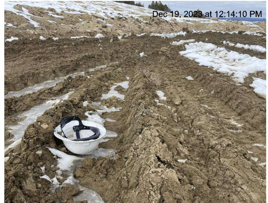
Photo # 217 Lack of stabilization/compaction/insufficient BMP's
