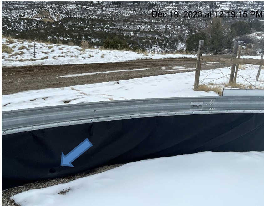
Photo # 198 Hole in liner/liner needs maintenance
