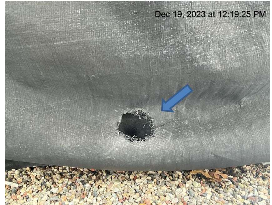
Photo # 199 Hole in liner/liner needs maintenance
