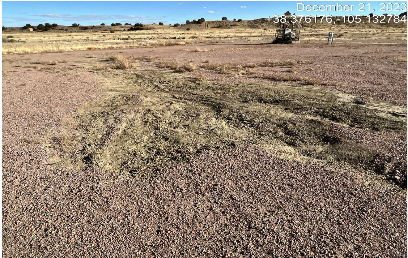
Photo 2. Facing east by the separator. The There was an attempt to repair the erosion however this area needs to be properly stabilized.
