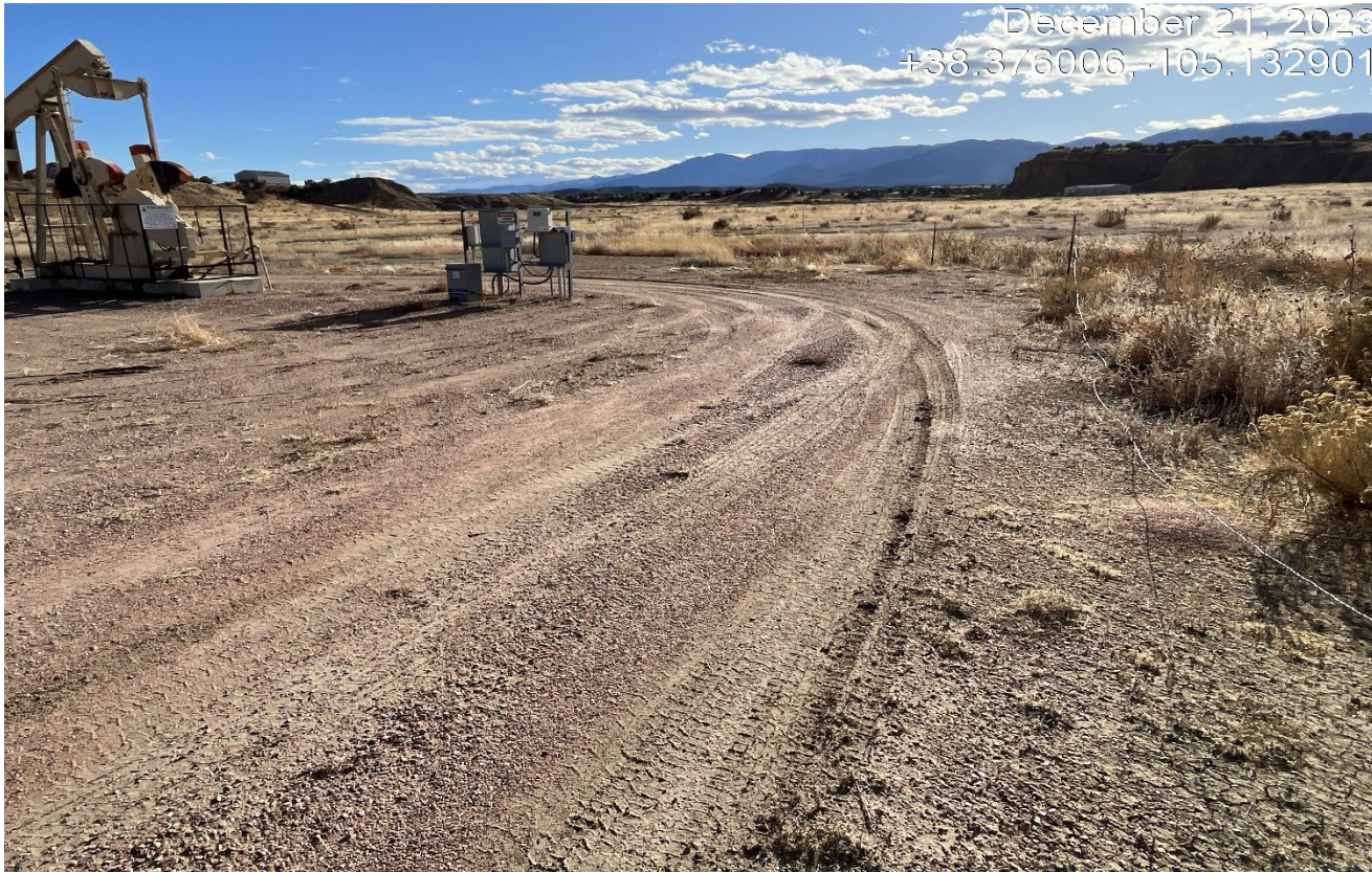
Photo 3. Facing southeast at west side of the location. The perimeter one wire fence is not maintained and needs to be removed or a proper fence installed.
