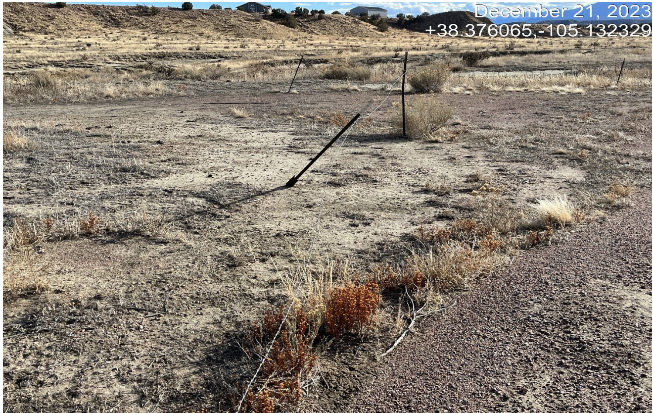
Photo 5. There is a one wire fence at the location which is not maintained and is not highly visible and could pose a collision hazard..
