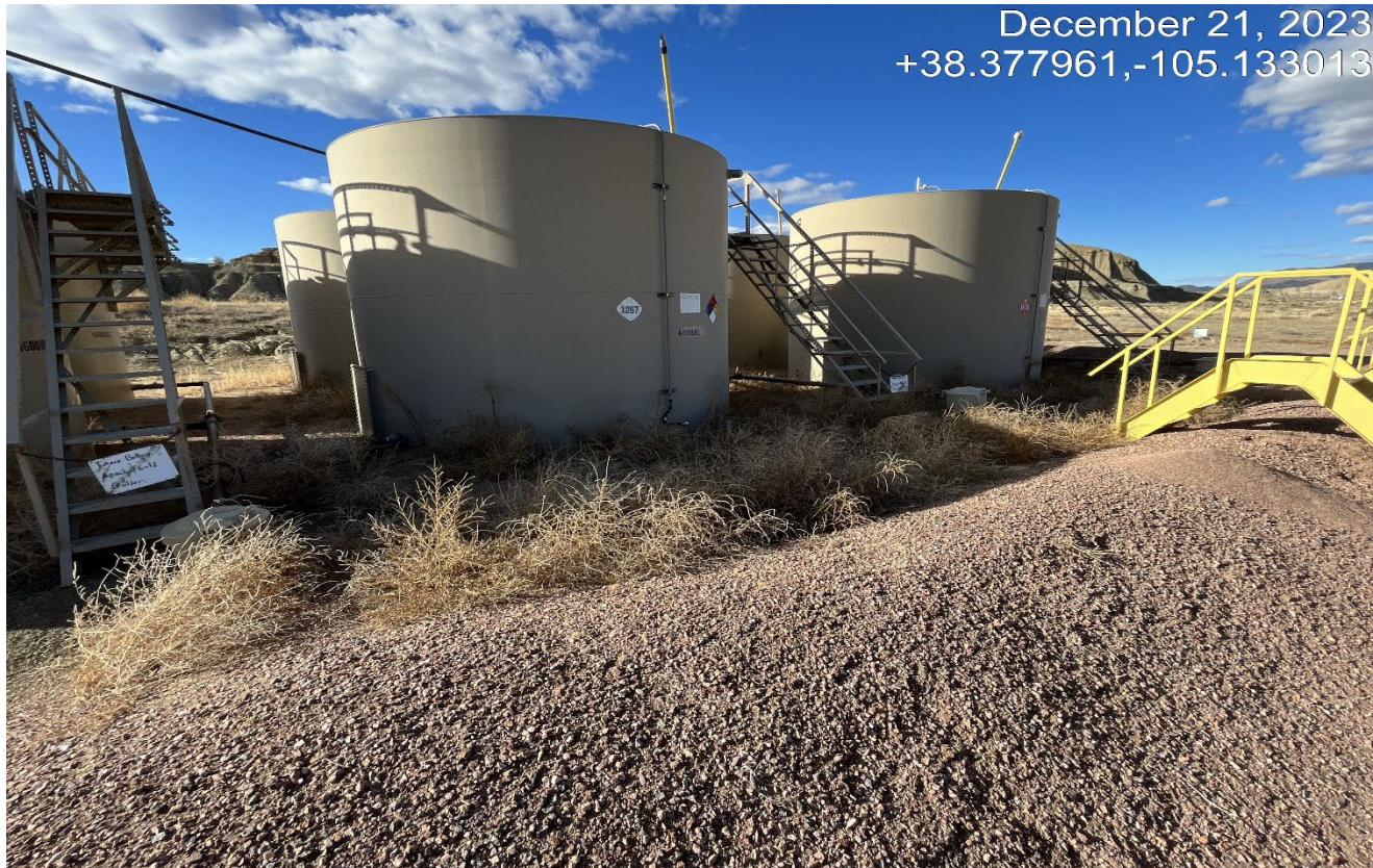
Photo 5. There are weed debris inside the tank battery that needs to be removed. There is not a proper sign posted at the tank battery.
