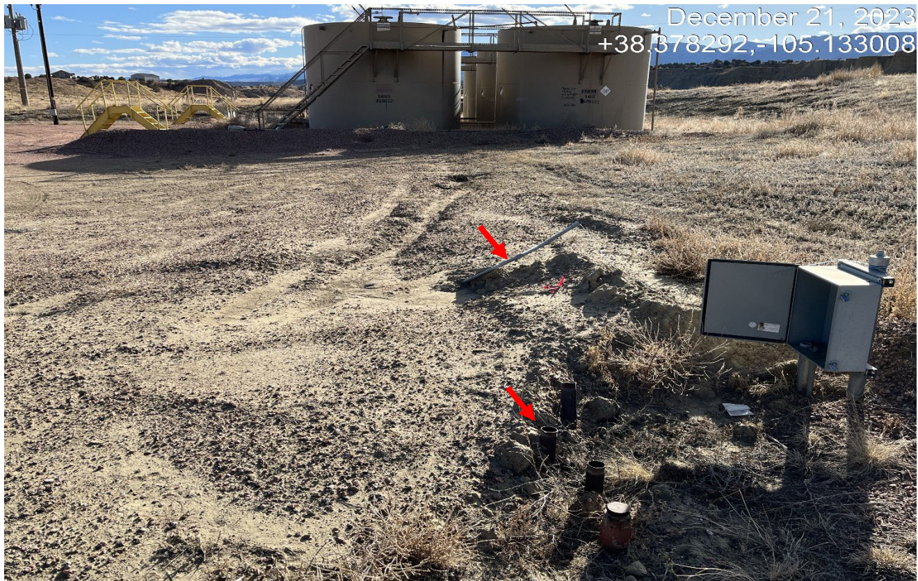
Photo 4. Facing south at the west side of the location. There is an exposed electric line at red arrow and multiple open pipe risers. All risers and utilities need to be removed.
