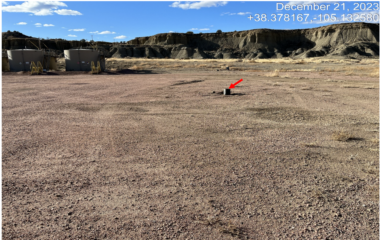
Photo 1. Facing west at the location. There is a plastic bucket covering an open wellbore at red arrow.
