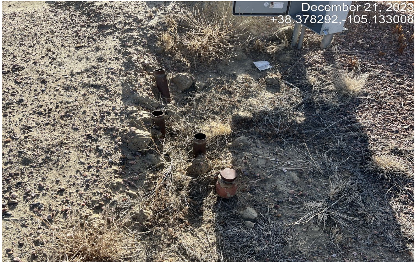
Photo 5. There are unused pipe risers that need to be abandoned and removed.
