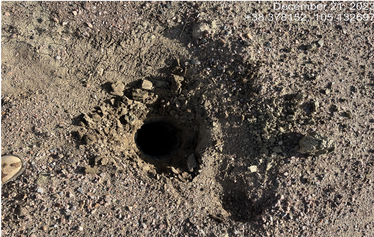
Photo 2. There is a well casing and deep wellbore which the plastic bucket was covering. This need to be immediately covered and plugged and abandoned..
