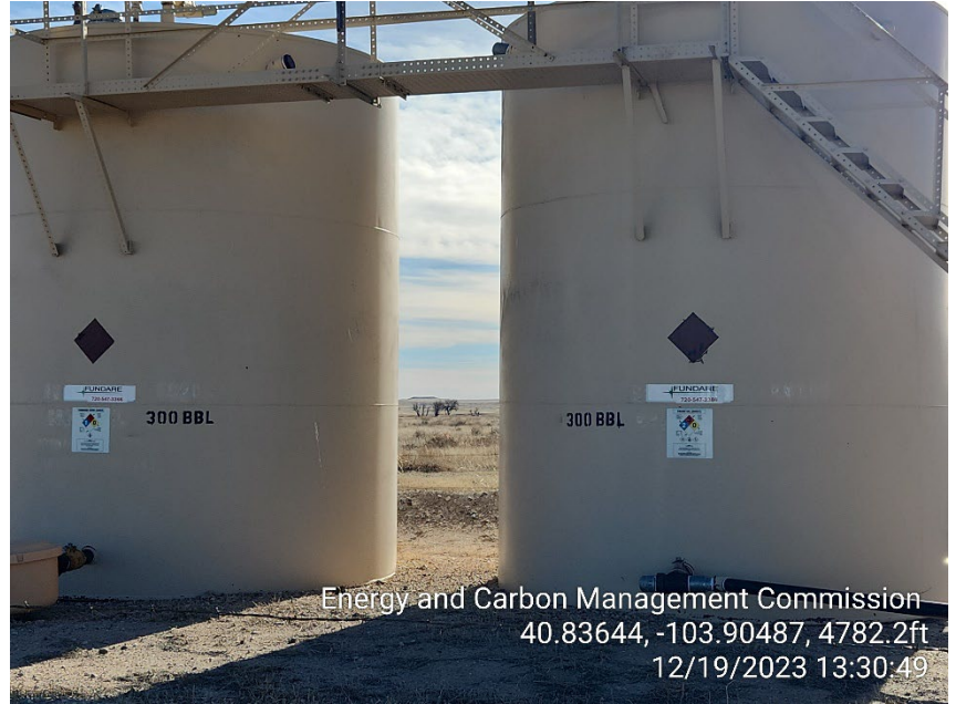
Photo 2 – Tank Battery
