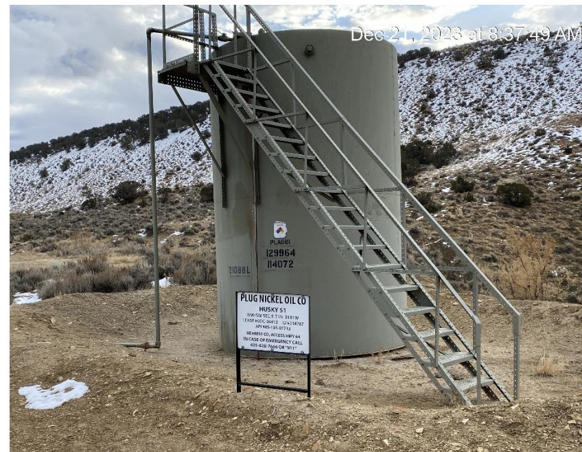
Undersize tank berm
