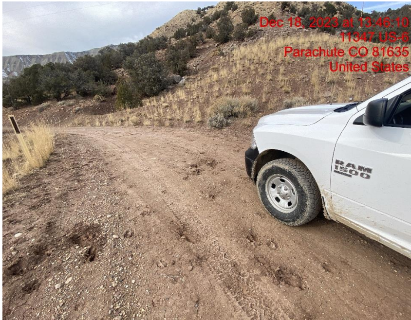
Insufficient Vehicle Tracking BMPs at Location Entrance/Exit – Photo #08286
