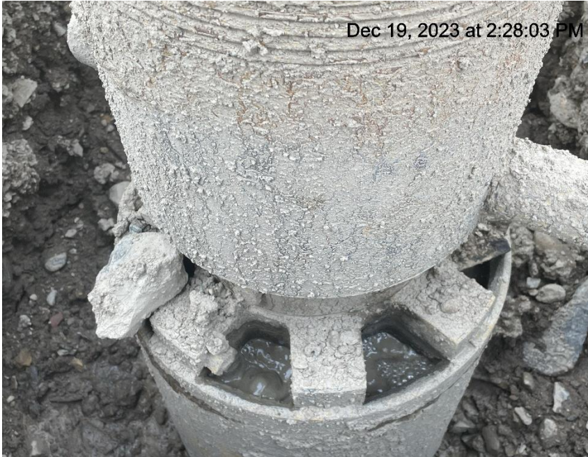
Photo # 397 Wellhead leak
